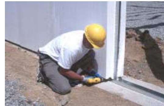
Panel is screwed into bottom track
