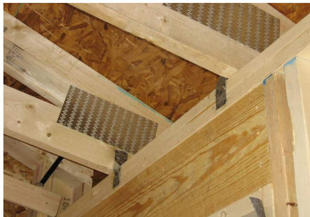
Panelized Wal Systems: Making the Connections
