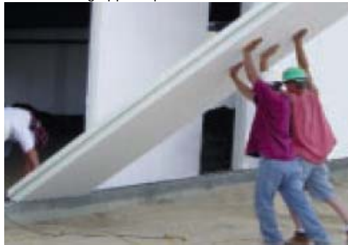
Panels being tipped up into bottom track
