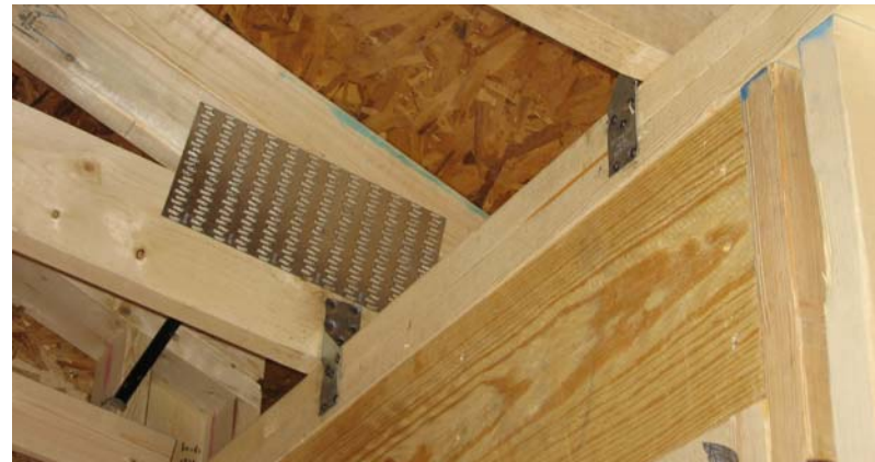
Wausau Homes panel/top plate connection interface
