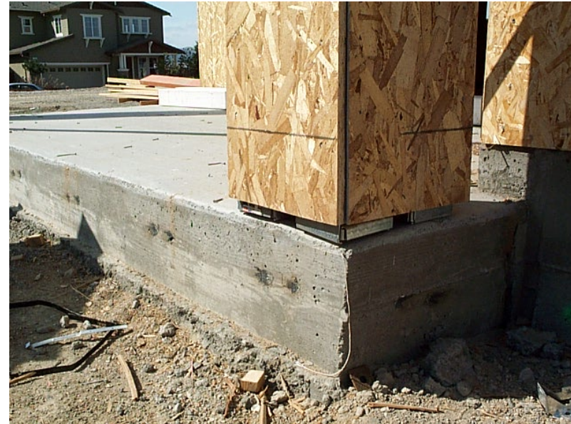
Panel/foundation connection point
