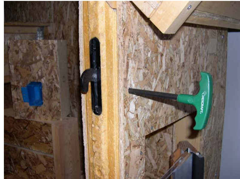
Murus Cam-Lock panel connection system
