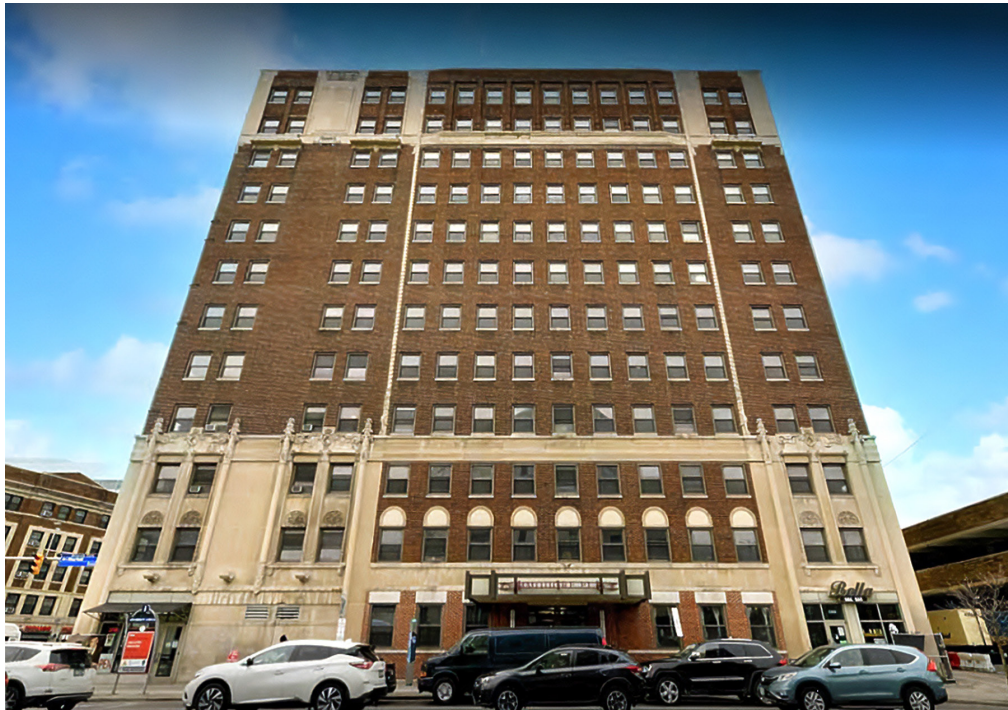
Front facade of Commodore Place Apartments after renovation. Photo credit: The Community Builders
