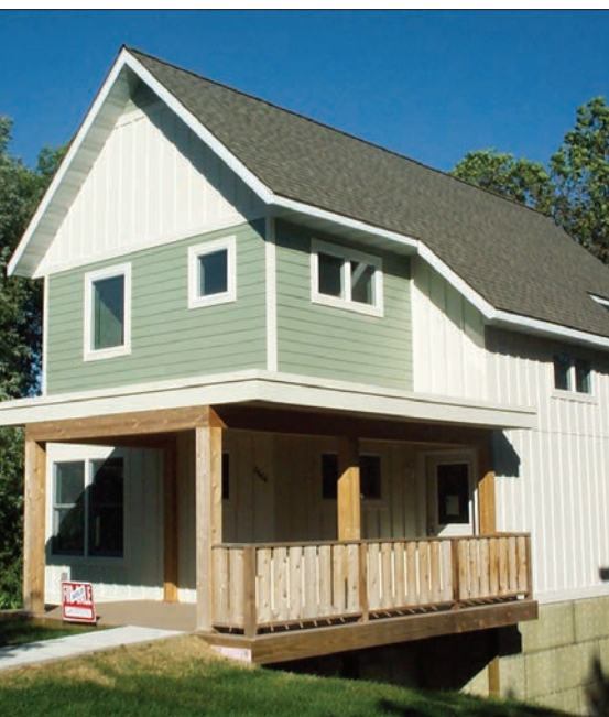
One Roof Community Housing was established by grassroots activists to provide affordable homeownership opportunities for residents of Duluth, Minnesota.
