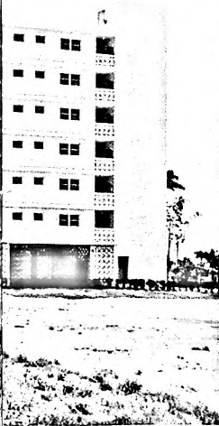
LEFT —Park Layne Towers in Hallandale, Fla., was the Nation's first HUD-FHA insured condominium apartment development.
