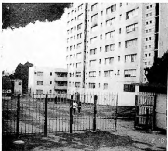
Courtyard between pairs of high rise structures, with gate and fence
