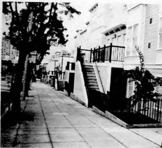
Street view, showing varying topography, cornice line, stair details
