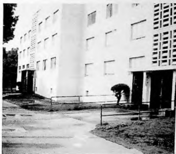
Low rise elements along sidewalk showing open entry stair
