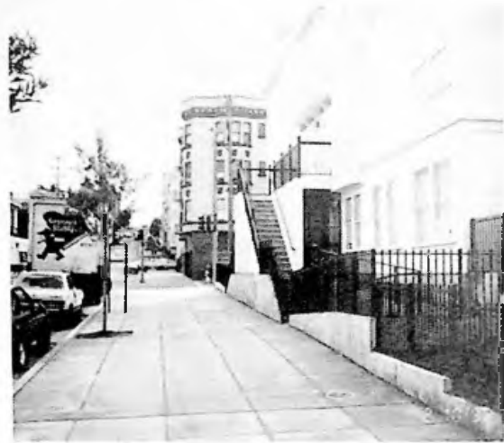
Street edge, showing relationship to adjacent housing on block beyond
