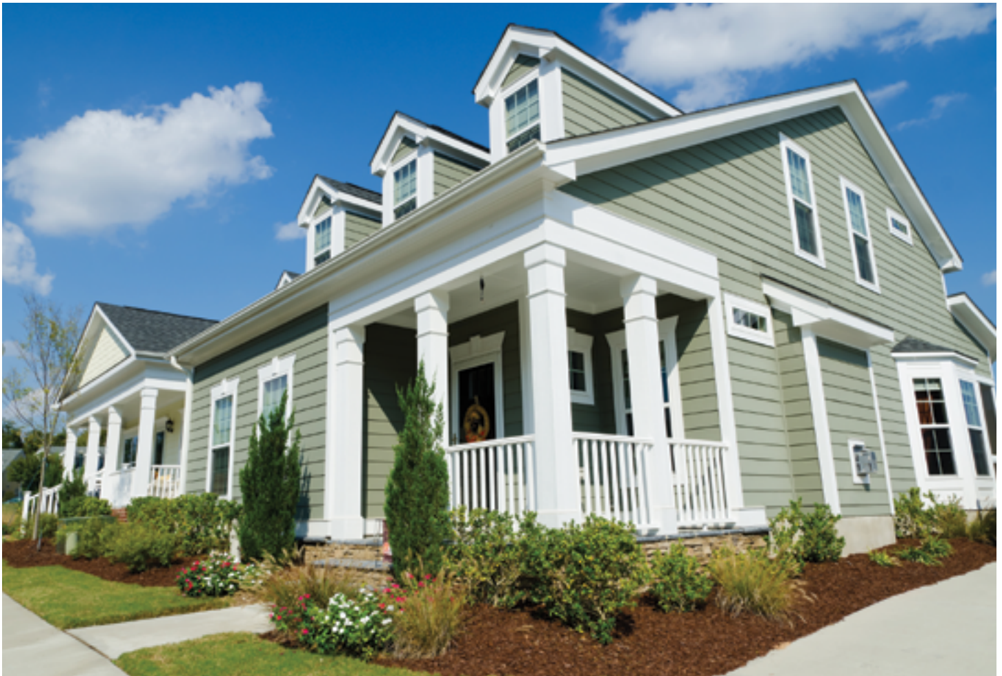
Higher density for single-family housing can be achieved through reduced setback requirements or zero lot line development.
