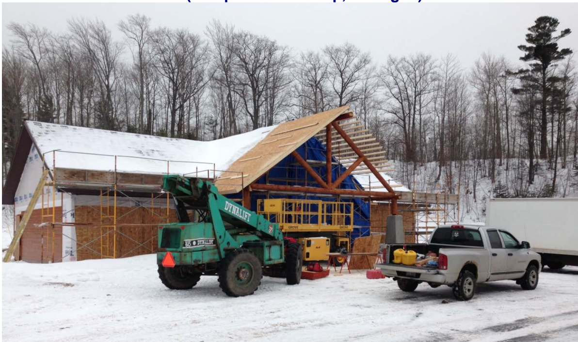
Figure 4: Keweenaw Bay Indian Community Travel Stop (Marquette Township, Michigan)
