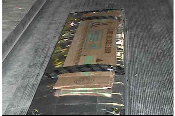
Cardboard spacer provides clearance for later saw cut through floor sheathing.
