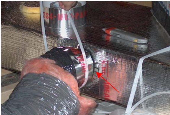
It is difficult to create a durable seal using tape or mastic alone.
