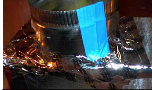
Round collars completely sealed with tape (above) or mastic (below) show no leakage.
