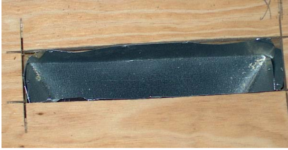
Perimeter supplies need to be sealed to the floor to prevent leakage into the belly.
