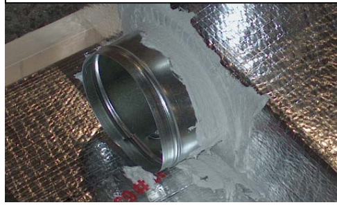
Round collars completely sealed with tape (above) or mastic (below) show no leakage.
