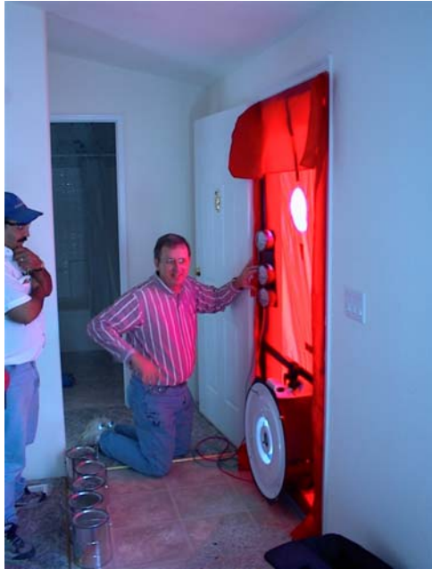
Blower door testing being conducted in a single section home outside the plant.
