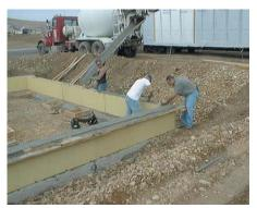
**Figure 2.4** Recessing the foundation to a depth below the frost line.
