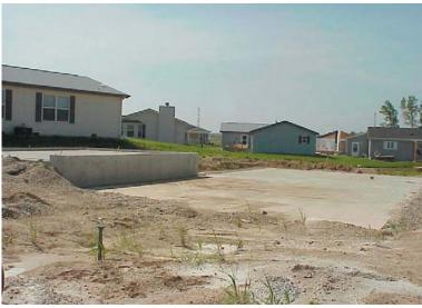
**Figure 3.51** Side-by-side slabs for a house and garage. The elevated garage foundation will keep the house and garage floors near each other vertically.
