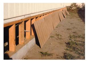
Figure 3.15 Ponywall construction method.
