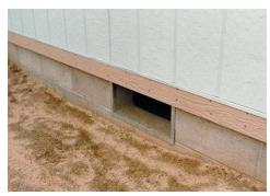
**Figure 2.10** Foundation wall detail showing an air vent.
