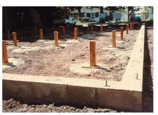
**Figure 3.16** Carefully placed anchor bolts will not interfere with any portion of the manufactured home's floor joists.
