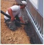
Figure 4.12 Concrete added to the trench.
