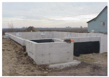
Figure 3.63 Basement showing backfill to create drainage slope.
