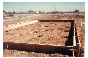
Figure 3.14 Forms ready for concrete pour.
