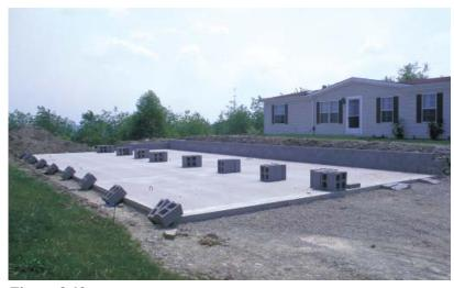
**Figure 3.46** The simple design of slabs minimizes the time required for fork work and provides a level base for the home.
