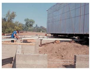
Figure 3.18 Installing a home with a roller system.
