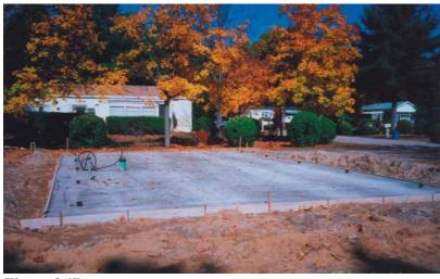
**Figure 3.47** Slabs provide a monolithic structural base that if uninsulated can move with shifting soil pressures.
