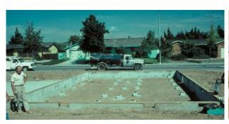
**Figure 3.10** A crawl space foundation system with full perimeter support, ready for home installation.
