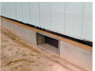
**Figure 3.21** The dark horizontal area is the manufactured home floor joist, covered with the bottom board. The light wood is the foundation sill. A factory installed flashing is visible at the bottom edge of the exterior siding.
