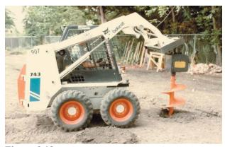
**Figure 3.13** Digging chassis support footers with a power auger.
