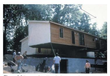
Figure 1.1 Crane set of a multi-section home on to a basement.
