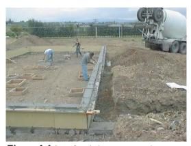
**Figure 1.4** Some foundations are recessed to create a "site-built" look.
