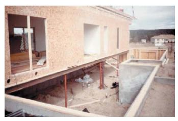
**Figure 3.68** The structure of the basement includes supports for carrying the home at the perimeter and centerline.
