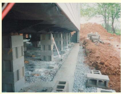
**Figure 3.27** Concrete block piers support the chassis I-beams. Anchors are encased in the concrete runners.
