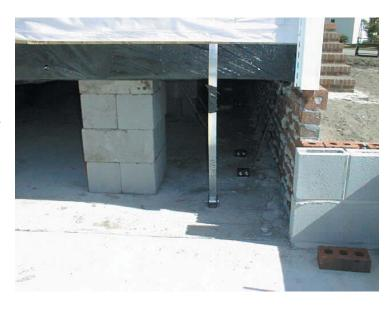
**Figure 3.49** This view under a home shows block chassis supports, embedded anchors, and masonry exterior wall.
