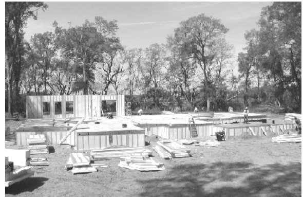
b. Sheathed floor platform and first set of panels
