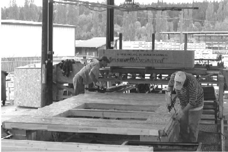
Figure 18 Application of Sheathing Panels
