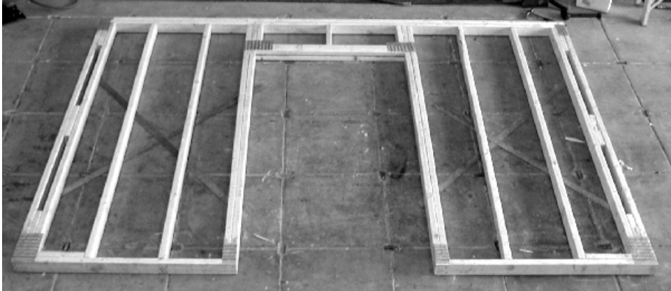
Figure 27 Wall Framing with Truss Plates
