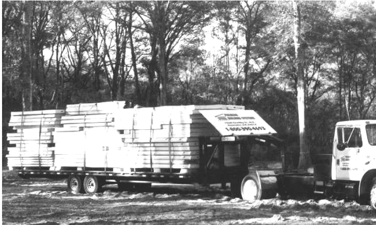
Figure 5 Transportation of the Wall Panels by Trailer
