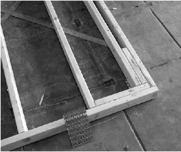
A. Before Plate Installation
