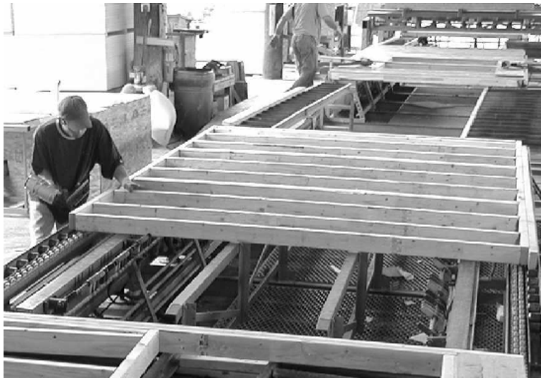
Figure 17 Wall Panel Being Framed
