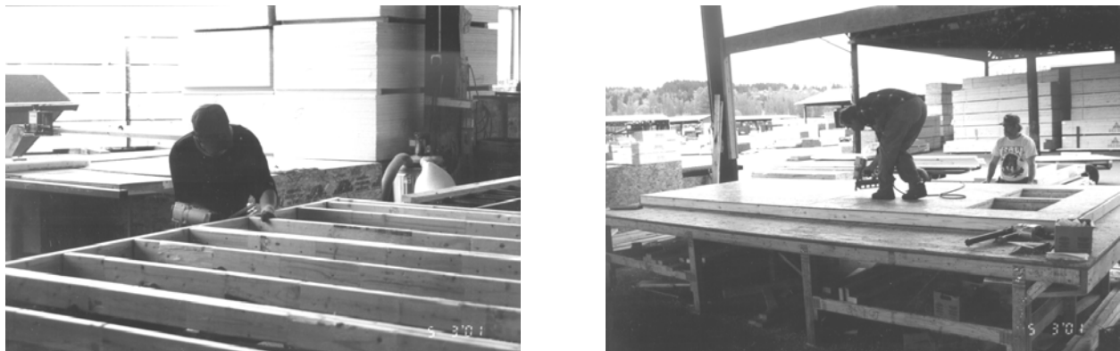
Figure 14 Fabrication of Light-Frame Wall Panels
