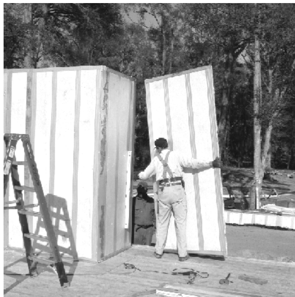
Figure 6 Panel Installation
