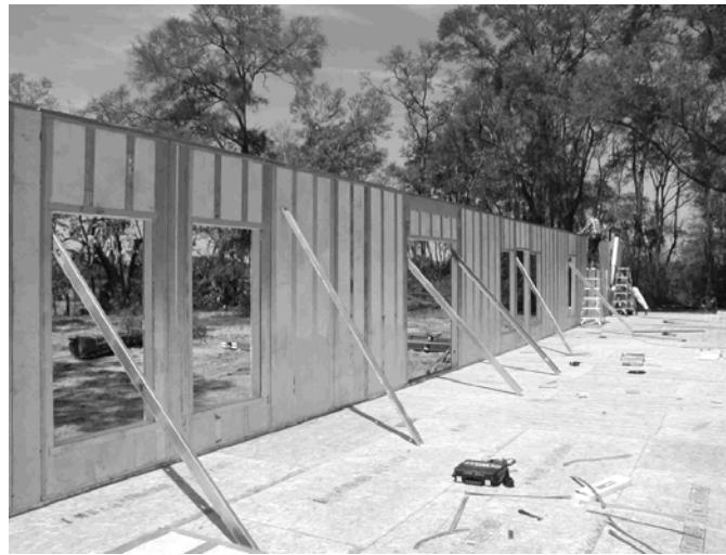
Figure 7 Wall Bracing
