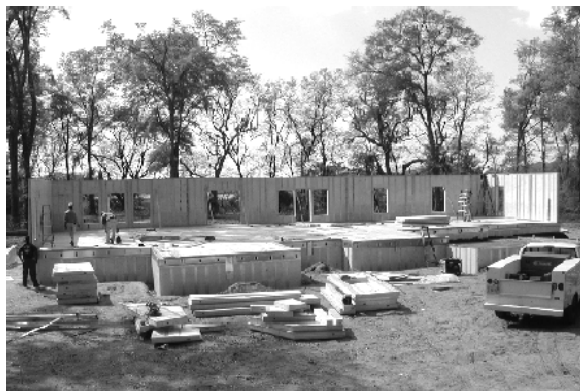
c. North, East, and West walls completed
