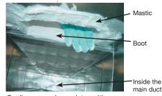
Sealing around a register with duct mastic -view from inside the duct
