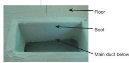
Boot sealed with mesh tape and mastic
