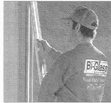
EXISTING SASH REMOVED, CAVITIES INSULATED AND NEW TRACKS INSTALLED
