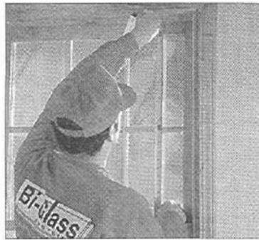
EXISTING WINDOW MEASURED AND GLASS UNITS FABRICATED
