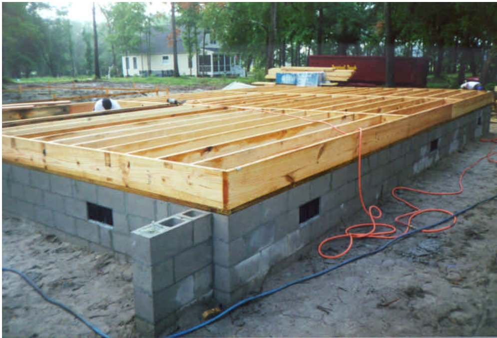
Wood House Floor Framing
