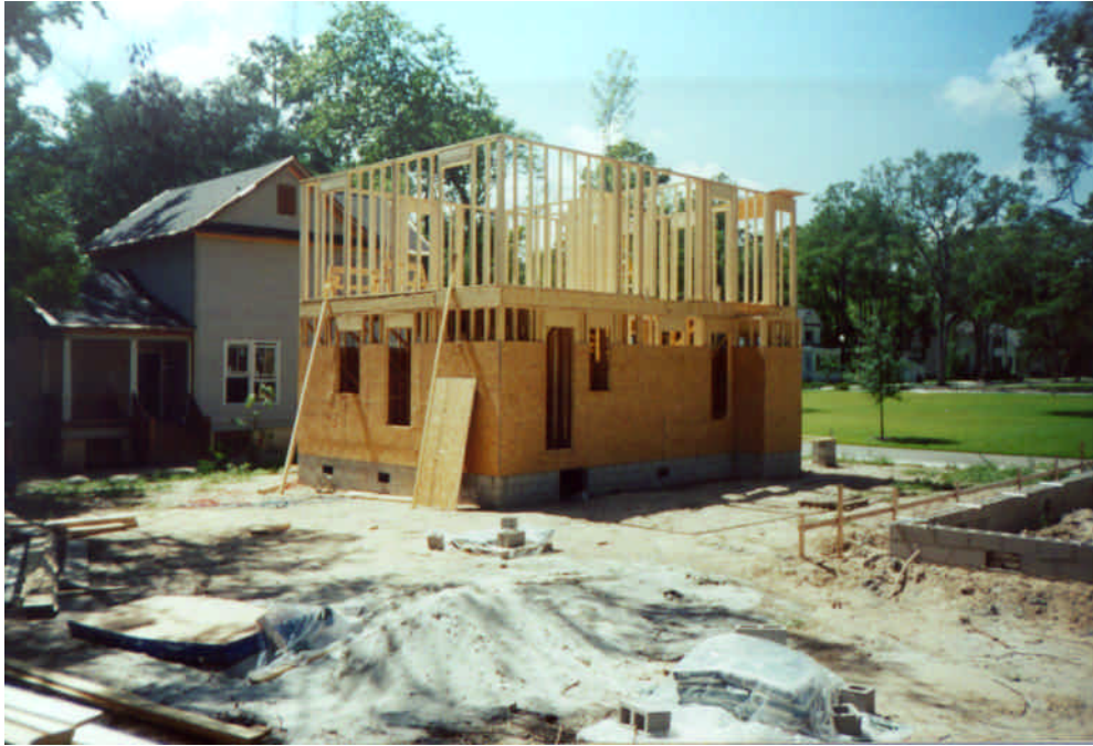
Wood House Wall Framing
