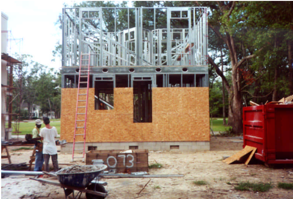
Steel House Wall Framing
