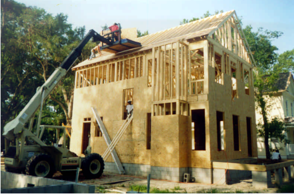
Wood House Wall Framing
