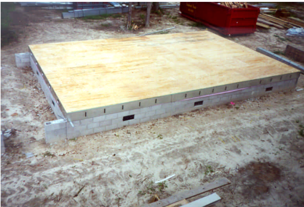
Wood House Floor Framing
