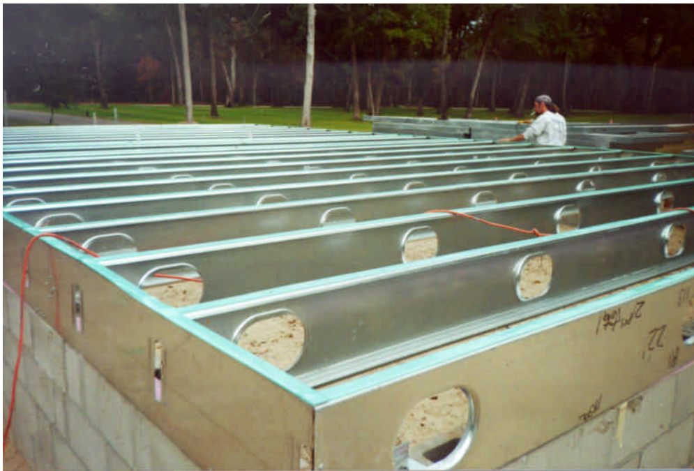
Steel House Floor Framing
