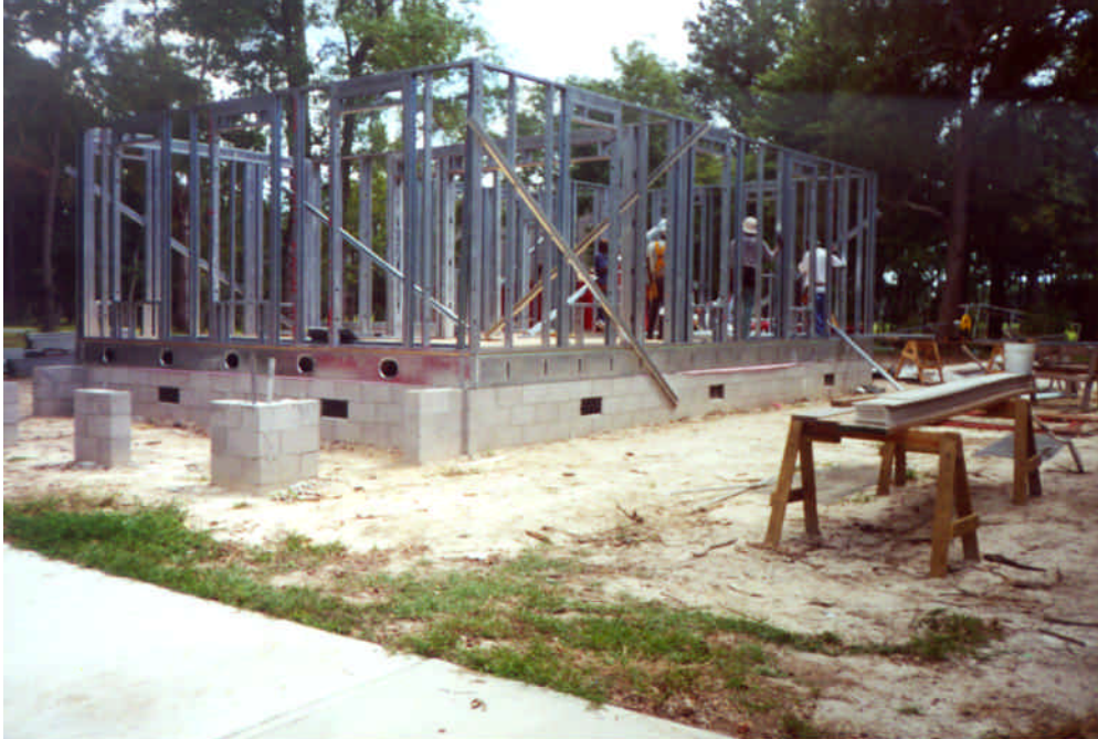
Steel House Wall Framing
