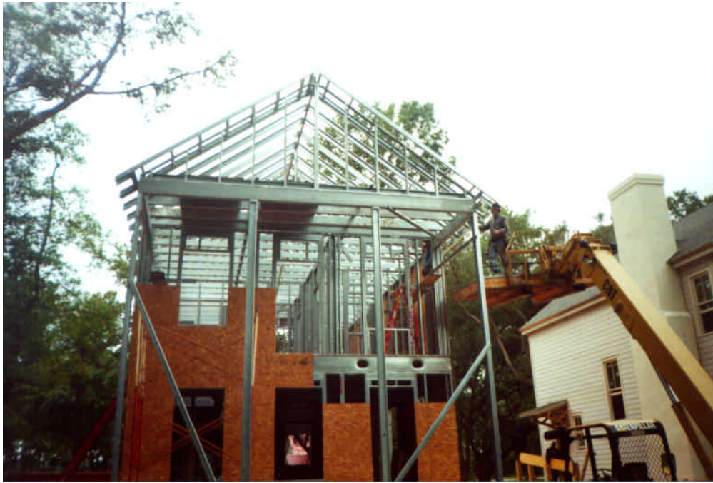
Steel House Roof Framing
