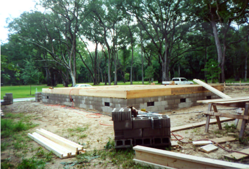
Wood House Floor Framing
