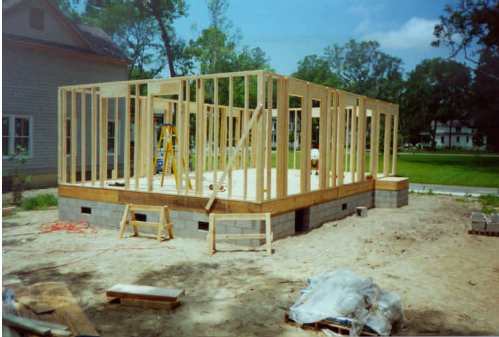
Wood House Wall Framing
