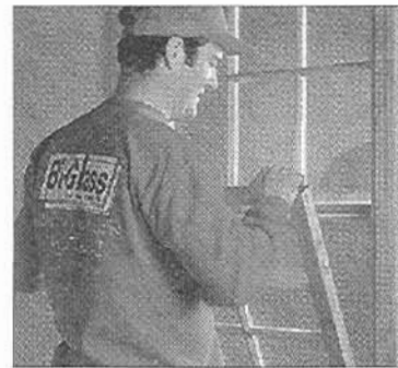
SASH IS INSTALLED WITH NEW HARDWARE PROVIDING FOR TILT-IN OPERATION
