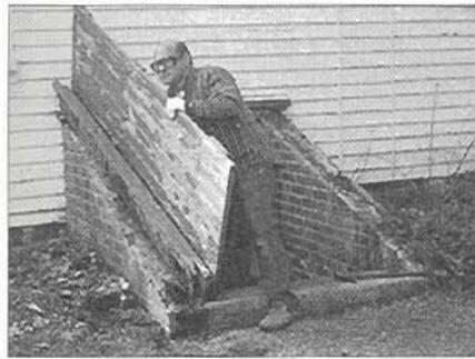
REMOVE OLD DOORS
