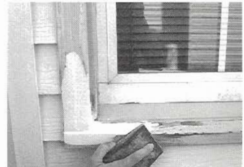
EPOXY FILLER APPLIED AND SANDED
