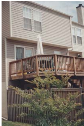
Figure 54 Example of a wood deck in good condition (1990s house sample).
