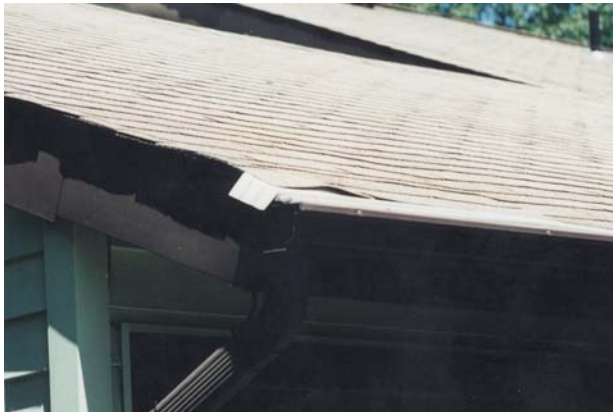
Figure 46 Example of a 1970s house sample with roofing rated as adequate.
