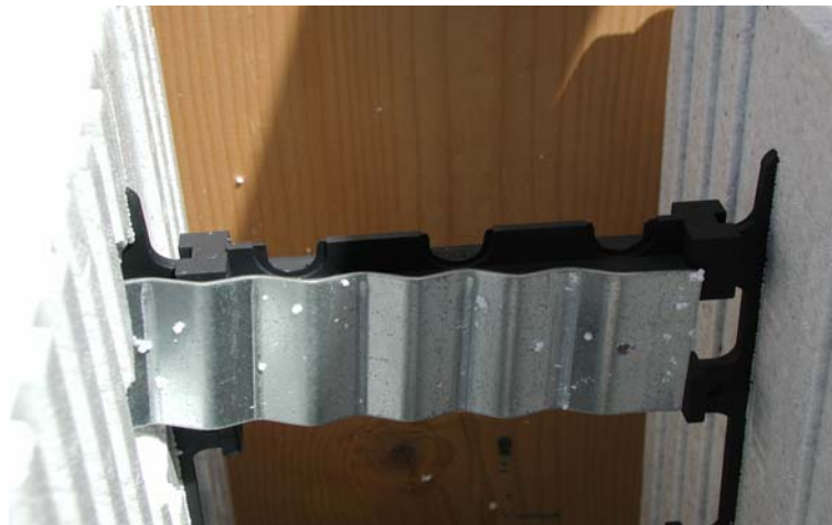
Figure 3 Richmond F-32 Anchor Installed in an ICF Form (face of anchor is flush with outside of form).
