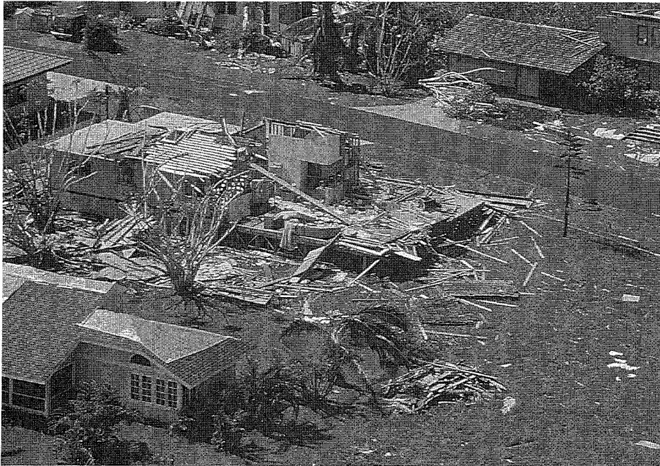
Figure 105. This home was struck by the roof blown off a neighboring home.
