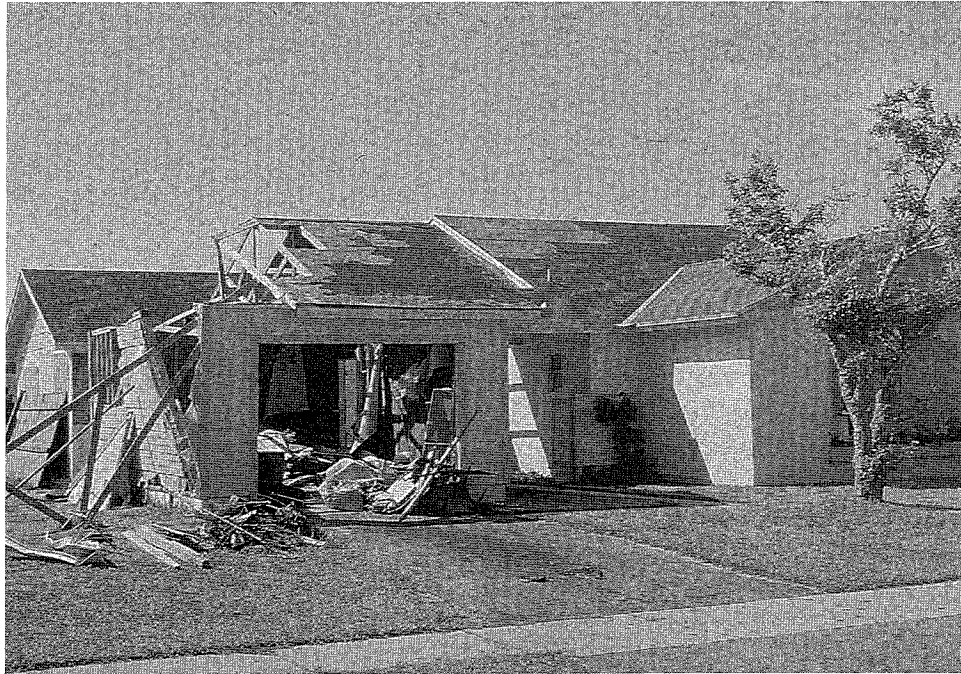
Figure 41. This garage door failure lead to internal pressures that contributed to blowing out the roof and the improperly connected wall corner joint of the garage.
