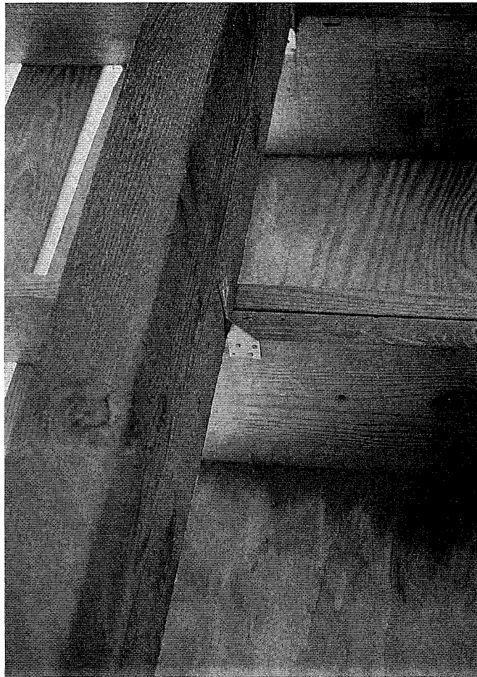
Figure 55. A small twist strap (six 6d nails total) was used to tie the floor joist to the foundation girder in this coastal home.
