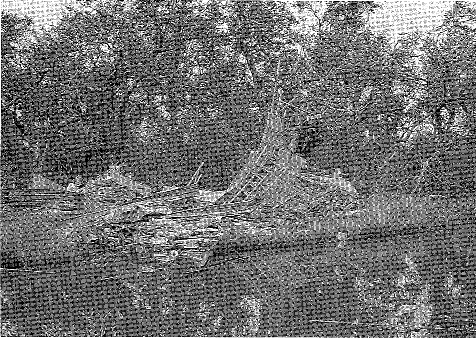
Figure 53. Upper story and roof of the home shown in Figure 52 (50+ yards downwind).
