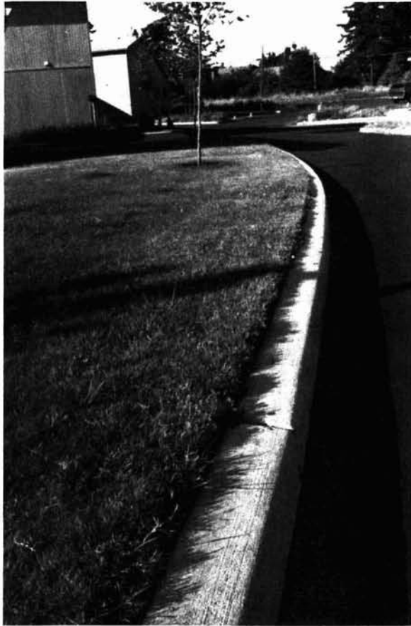
Vertical curb without gutter
