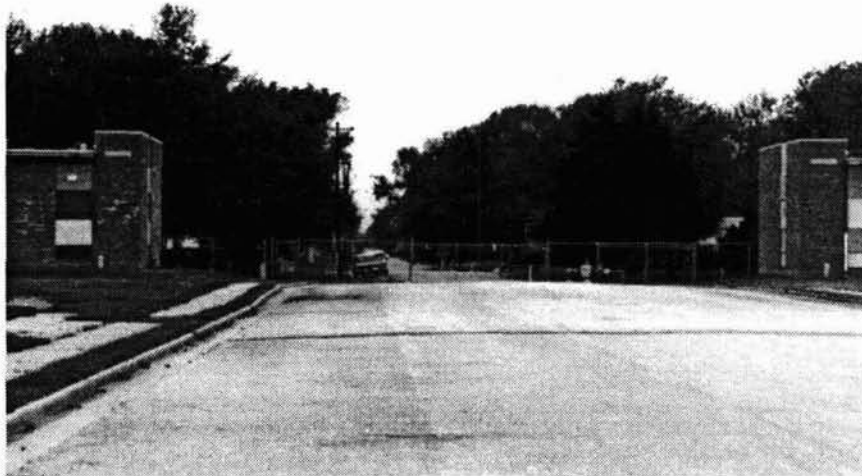
Photo 2.2 Worsening crime led to the erection of fencing limiting access to the property. (Carole Walker)
