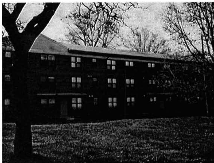
Photo 1.3 Cherry Hill public housing after modernization. (David Varady)
