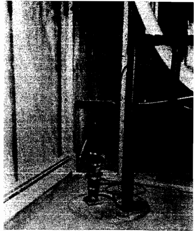
Septic system hook-up
