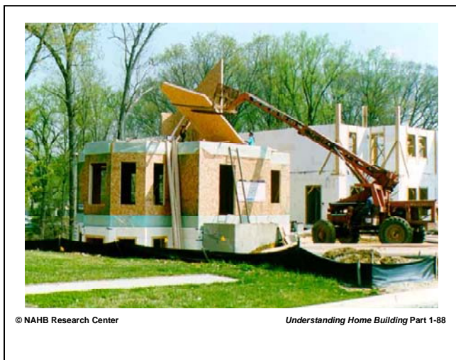
Figure 2-5: Structural insulated panels being installed
