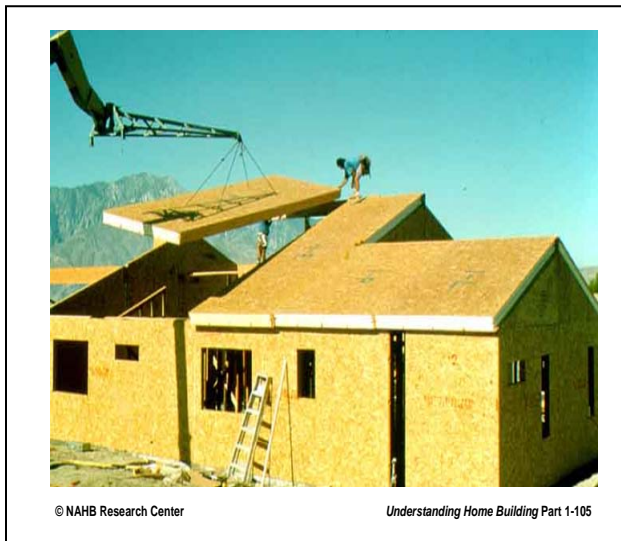
Figure 2-4: Structural insulated roofing panel
