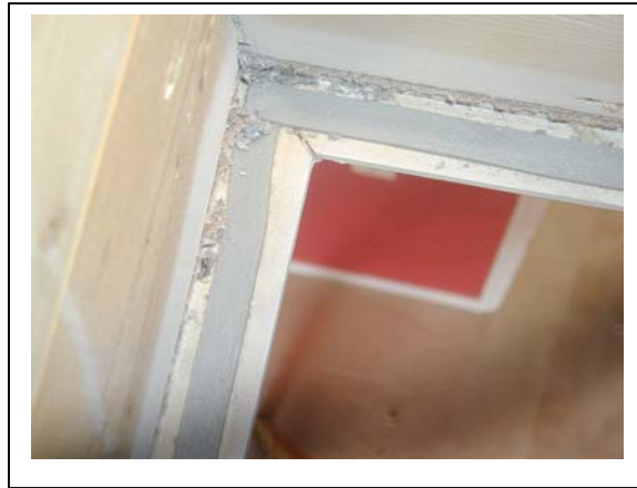
Figure 15 Gasket in Place
