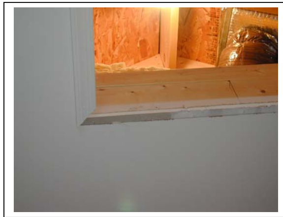
Figure 13 Attic Hatch Opening
