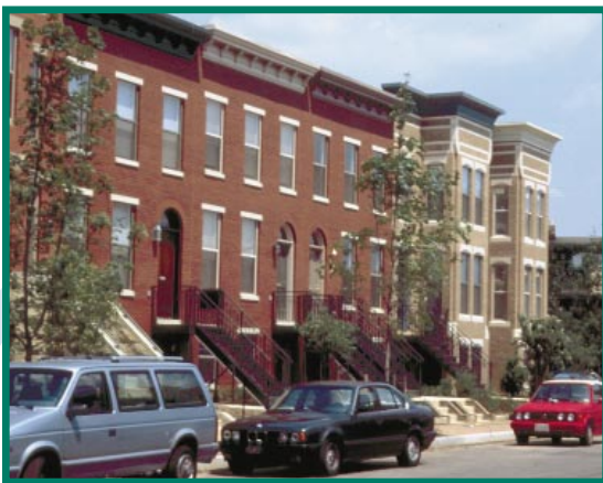
The former Ellen Wilson Dwellings has been rebuilt as a mixed-income cooperative, Washington, D.C.
