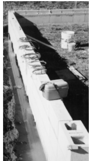
Figure 5 – CMU Foundation Wall
