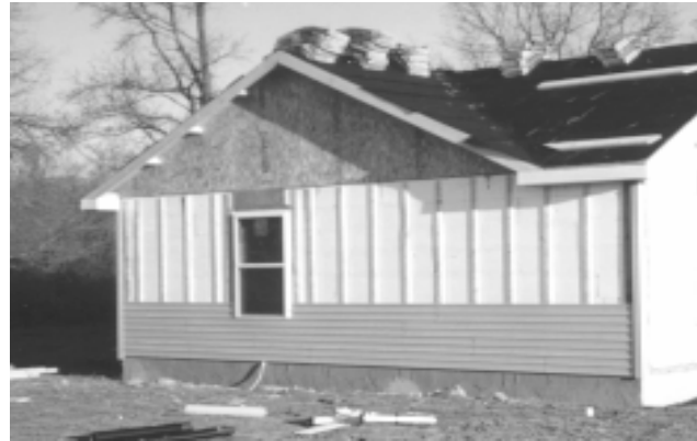
Figure 9 - Vinyl Siding on Reddi-Form House
