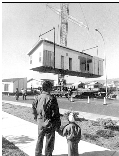
Figure 2.1: Manufactured housing is transferred to the construction site and lowered onto its foundation Source: HUD
