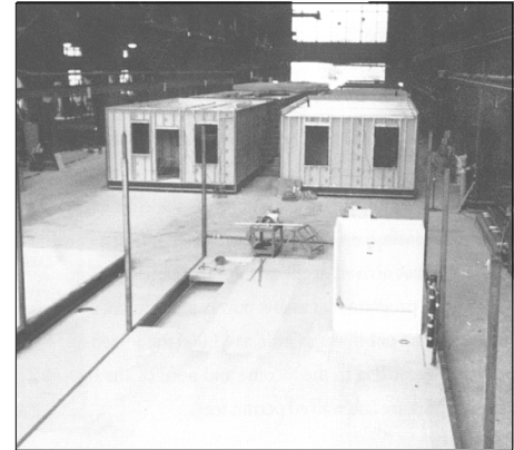
Figure 2.2: Modular housing on the factory floor Source: HUD
