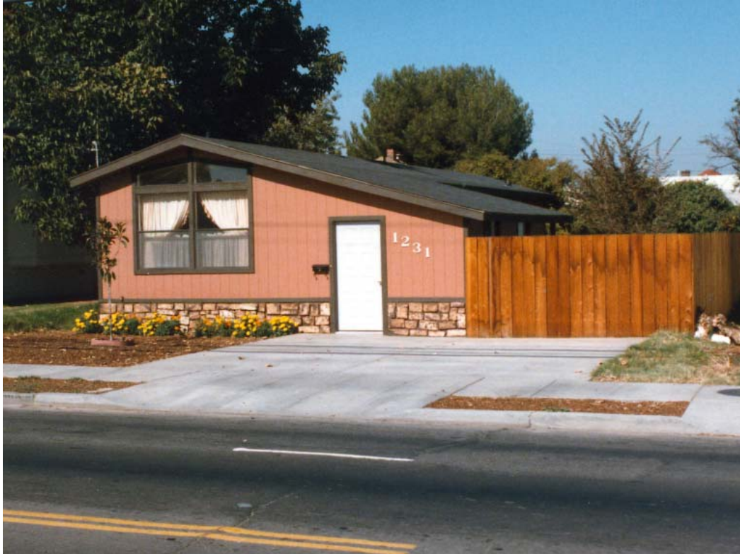
Figure 2.9: Early Attempt to Get Rid of the Singlewide Look by Extending Roof
