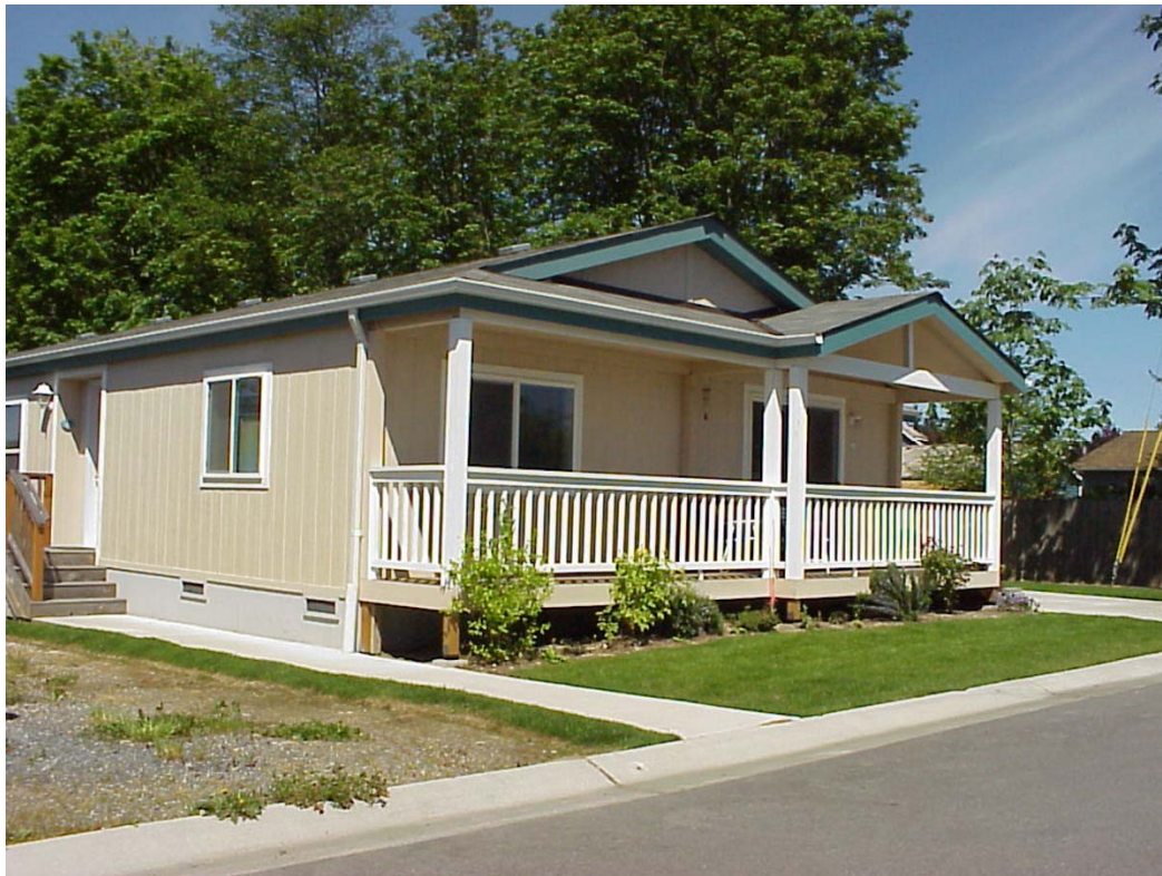
Figure 3.7: Manufactured Home in Thomas Place, Everett, Washington
