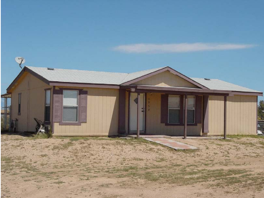
Figure 4.1: Typical Manufactured Home in Rural Pima County
