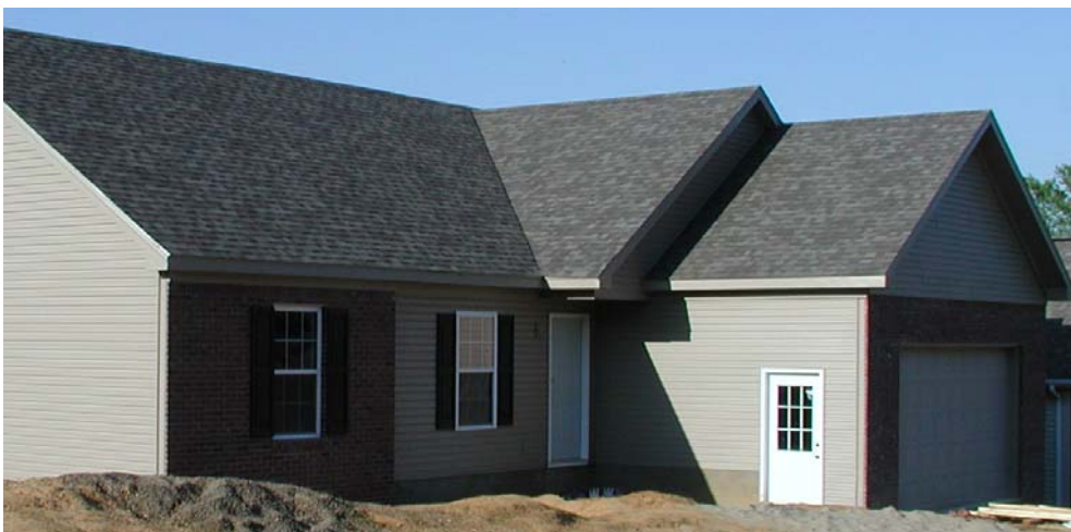
Figure 5.6: One-story Site-built Home Under Construction with Attached Garage
