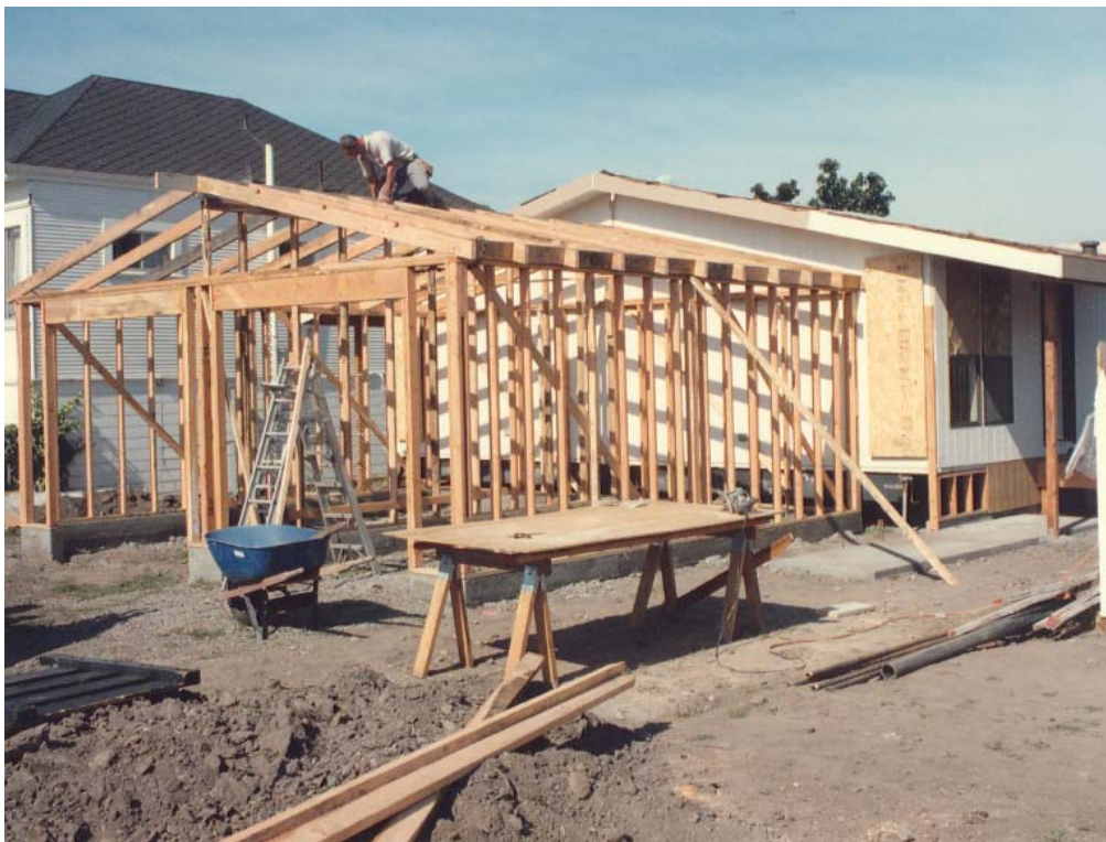
Figure 2.8: Garage Abutting Front of Manufactured Home
