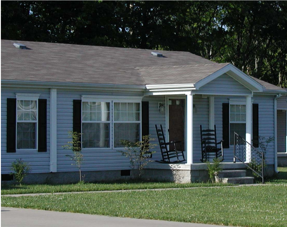
Figure 5.1: Manufactured Home With Post-production Porch, Vinyl Decorative Column, and Roof Vents (attributed to steeper pitch)
