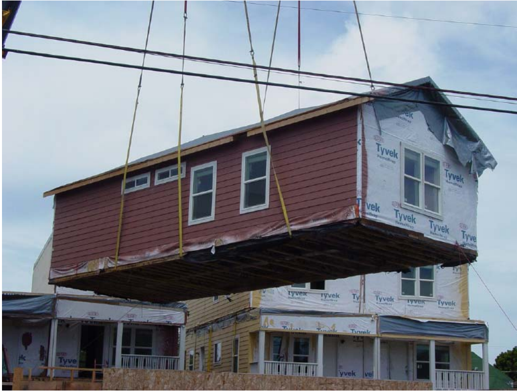
Figure 2.15: Crane Installation of HUD-Code Home
