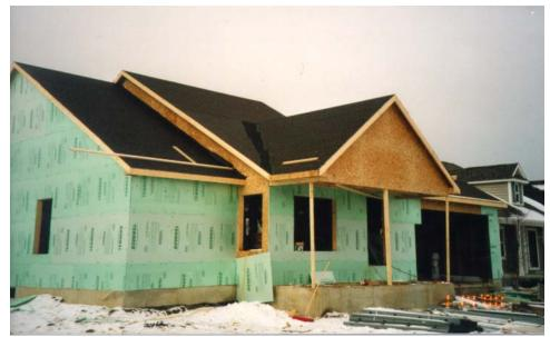
Steel House Sheathed with Rigid Foam Insulation
