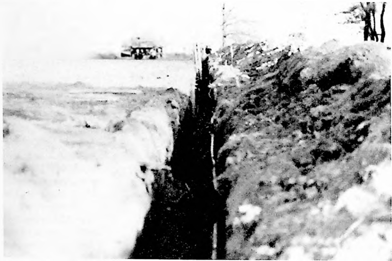
Common trench during site development work
