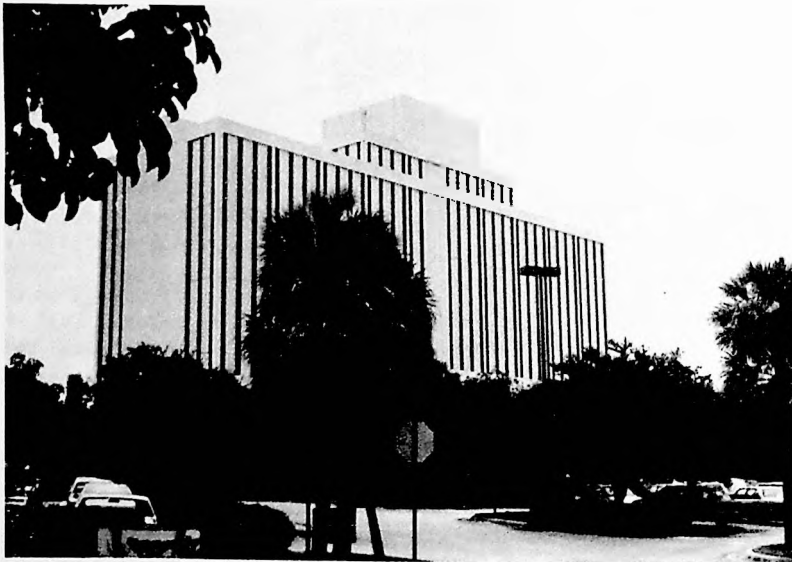
Coral Ridge Properties, Inc., main offices
