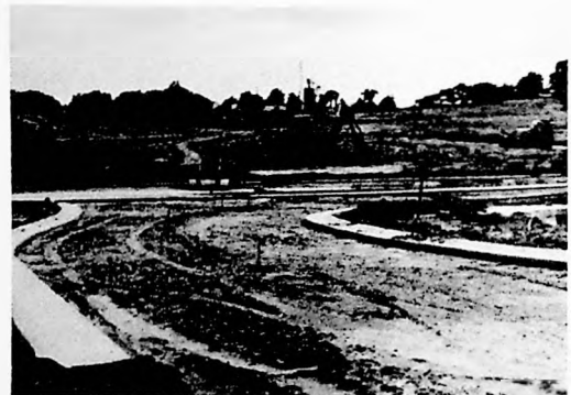
Woodland Hills roll curbs during construction
