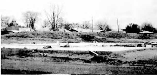
Slab-on grade foundation
