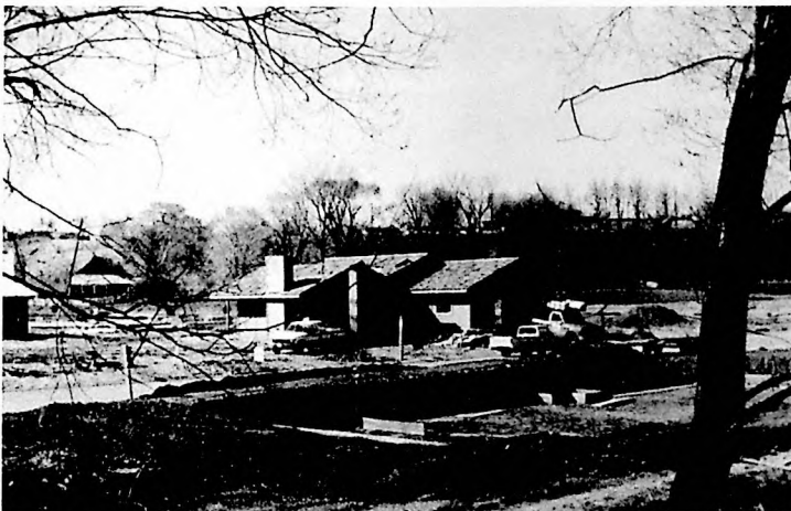
Lakewood Meadow unit under construction
