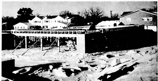
Eight-plex under construction
