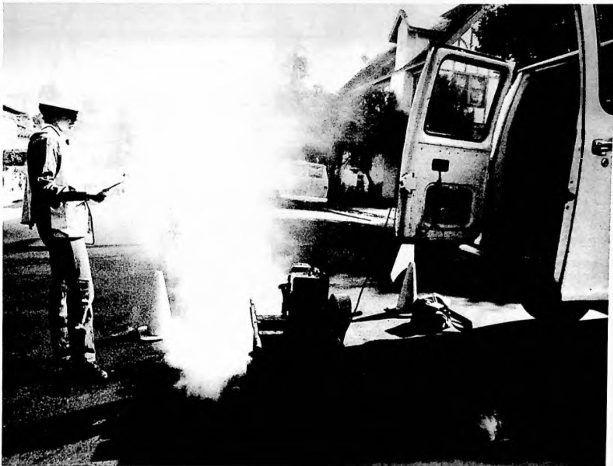
Figure 3-16 Field Engineer Prepares Smoke Test Blower Set-Up
