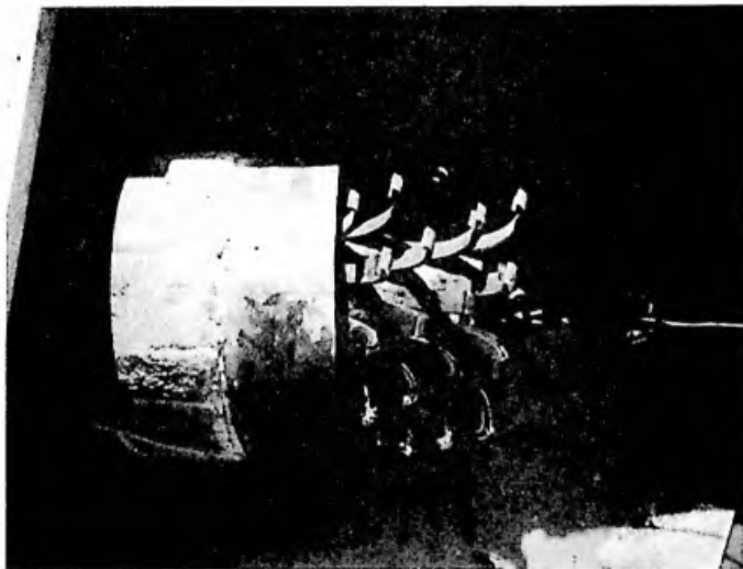
Figure 5-17 Mechanical Drag Cleaner Being Pulled Into Pipe. Courtesy of East Bay Municipal Utility District.
