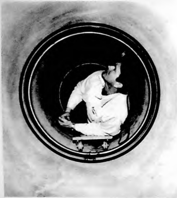
Figure 5-48 Weko-Seal Installation Being Inspected. Courtesy of Miller Pipeline Corporation.
