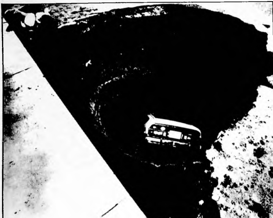
Figure 1-1 Newspaper Carrier's car lies in 30-foot-deep hole caused by leaking sewer. Courtesy Associated Press World Wide Photo
