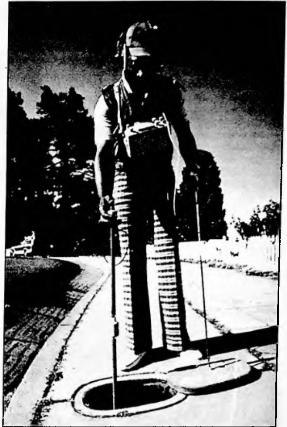
Figure 3-6 Sonic Leak Detection Equipment in Use. Courtesy of East Bay Municipal Utility District
