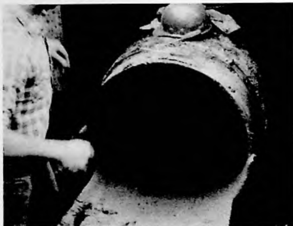
Figure 5-18 Cement Mortar Lining Machine in Pipe. Courtesy of East Bay Municipal Utility District
