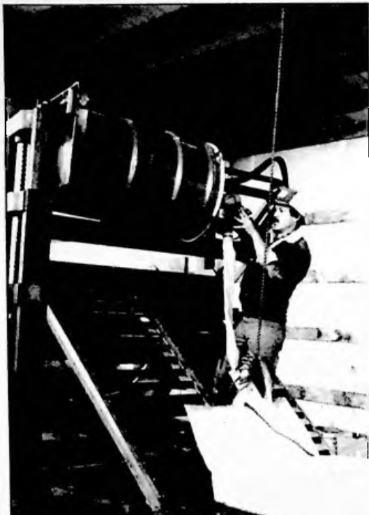
Figure 5-33 Insituform Felt Tube is "Wetted-Out" With Resin at Contractor's Shop
