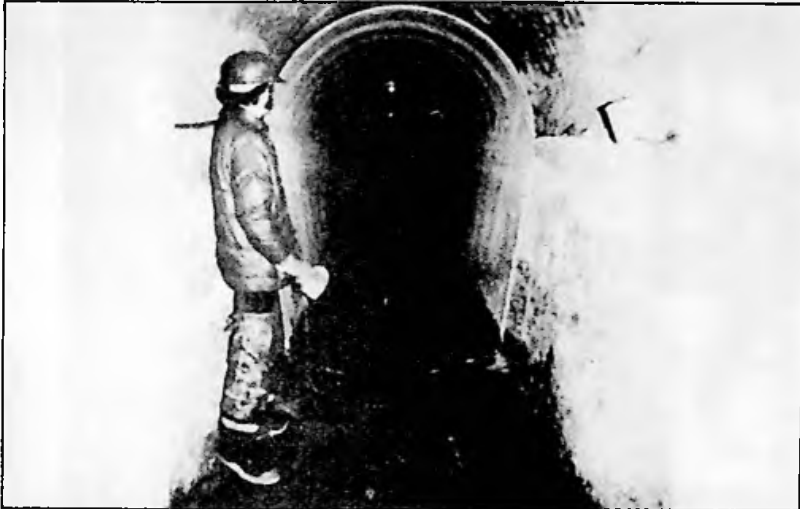
Figure 5-43 Segmented Fiberglass Reinforced Plastic Liners Can be Made in Many Shapes
