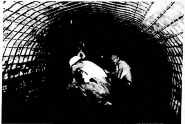
Figure 5-22 Reinforced Shotcrete Being Used to Rehabilitate a Large Diameter Brick Sewer
