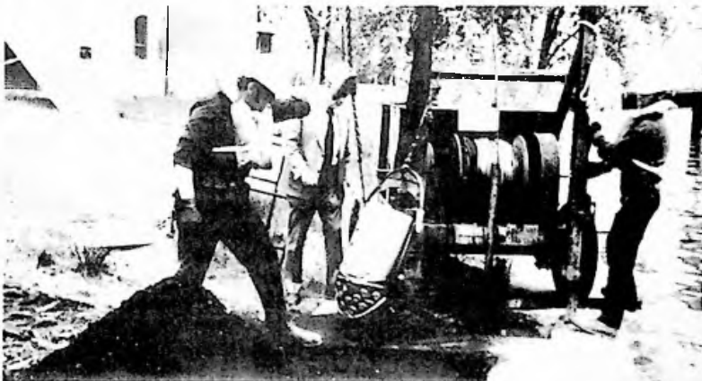
Figure 3-25 Bucket Machine Removes Loose Grit in Sewer. Courtesy Rodding-Cleaning Services, Inc.
