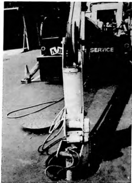
Figure 5-25 Modern Truck-Mounted Winch and Specially-Designed Boom Easily Pulled a 700-Foot, 24-Inch Polyethylene Liner in Less Than a Day
