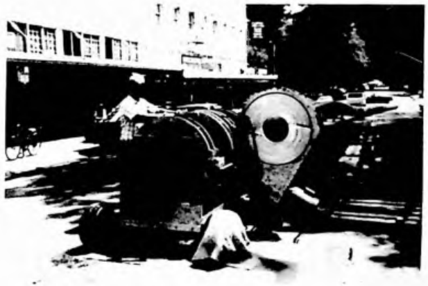
Figure 5-28 High Density Polyethylene Pipe is Heat Fused Into a Continuous Liner for Insertion by Slip Lining
