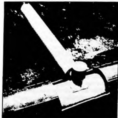
Figure 5-47 Reconnection of Gas Service Line. Courtesy of National Energy Leasing Company.
