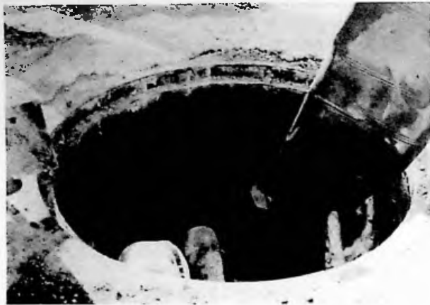
Figure 5-52 Placement of Joint Sealing Tape Between Manhole Frame and Cone Section
