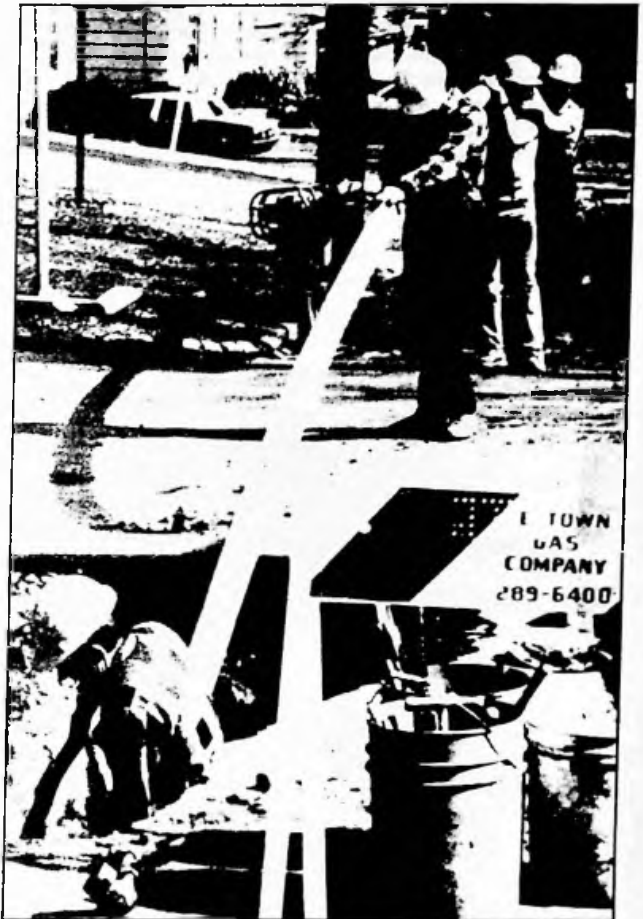
Figure 5-47 Reconnection of Gas Service Line. Courtesy of National Energy Leasing Company.
