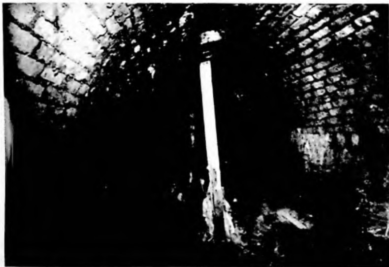
Figure 3-28 Sewer With Temporary Prop to Support Sagging Crown
