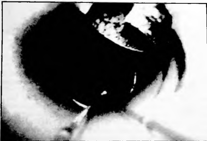
Figure 3-19 Protruding Sewer Lateral. Courtesy Rodding-Cleaning Services Inc.
