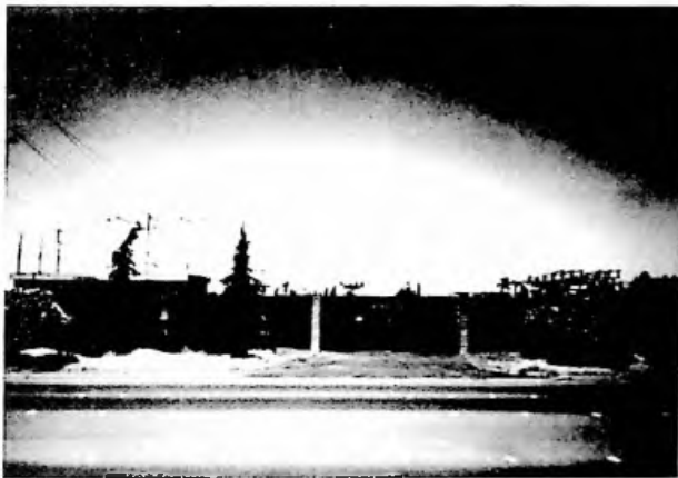
Figure 6-3 Examples of Electrical Substation--With and Without Visual Barrier. Courtesy Pacific Gas and Electric Company
