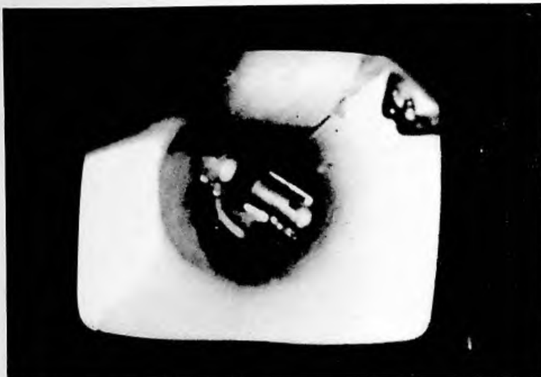
Figure 5-38 Insituform Remote Cutter Reconnecting a Service Lateral
