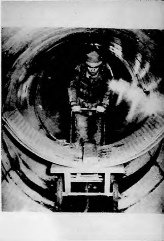
Figure 5-42 Segmented Fiberglass Reinforced Cement Liners are Easy to Handle
