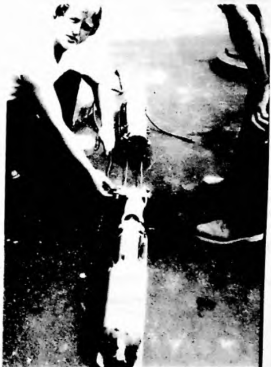
Figure 5-37 Insituform Cutter (foreground) and television camera (background)
