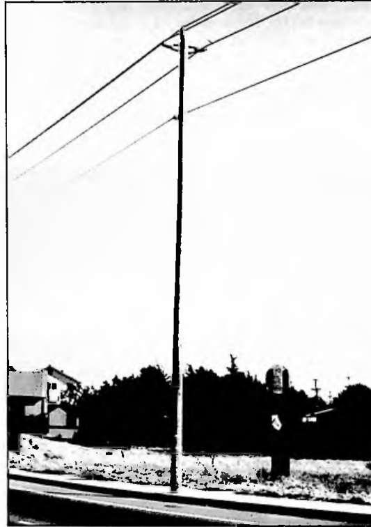
Figure 6-4 21-KV Distribution Line
