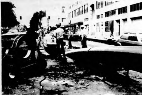
Figure 5-29 Polyethylene Liner is Pulled Into the Deteriorated Pipe at an Insertion Access Pit
