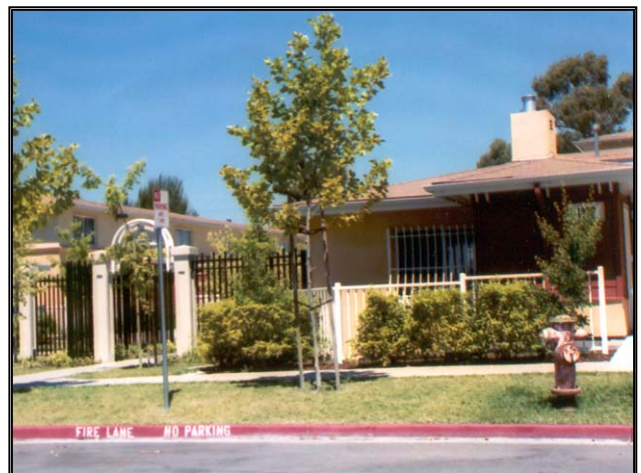
Figure 4-4. Rehabilitated unit at Lockwood Gardens.
