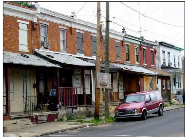
Figure 6-6. Boarded-up housing in the McGuire Gardens neighborhood.
