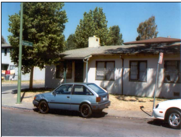
Figure 4-3. Unrehabilitated unit at Lockwood Gardens in Oakland.
