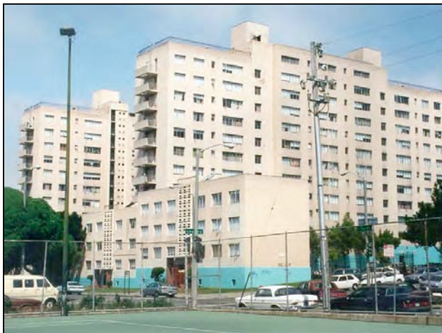
Figure 4-1. Plaza East in San Francisco prior to demolition.
