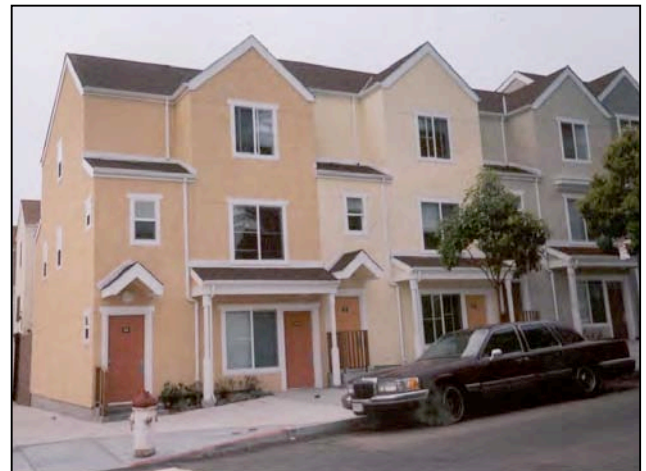
Figure 4-2. Redeveloped units at Plaza East.
