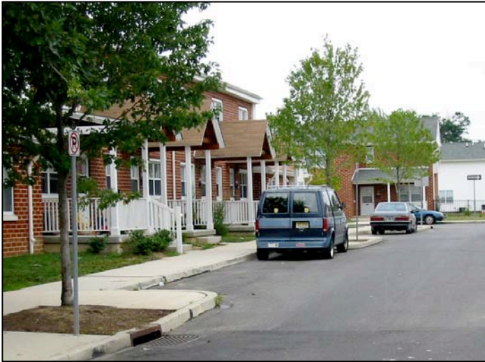
Figure 4-7. New through street and sidewalk at McGuire Gardens in Camden.
