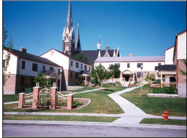
Figure 4-5. Rehabilitated units and courtyard at Hillside Terrace in Milwaukee.
