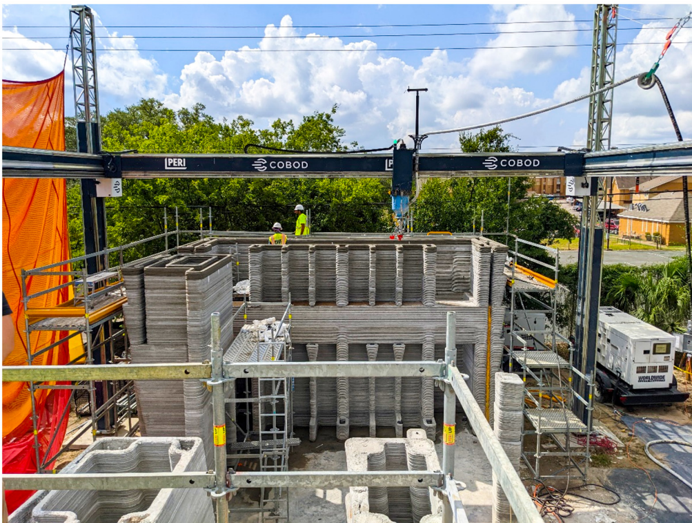
Note: 3D Printed Wall by PERI. Source: Home Innovation Research Labs
