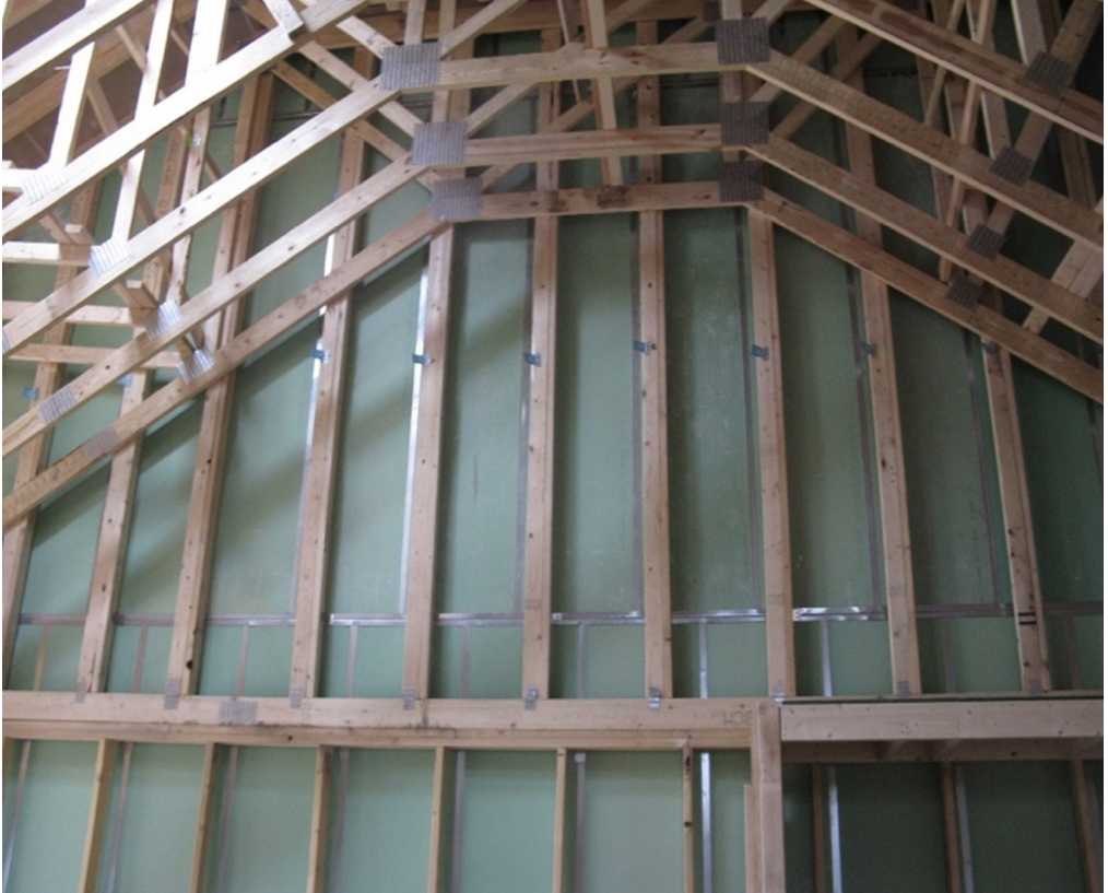
Example of a 2-hour fire-rated gypsum shaftliner assembly. Photo credit: Newport Partners.
