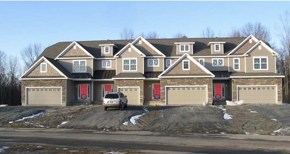
Guarded blower door testing, with a blower door on the doorway of each townhome, is expensive and impractical, because construction on the entire building must be temporarily halted. Photo credit: Newport Partners.
