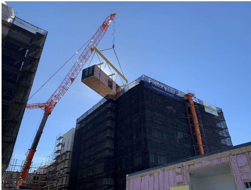
Modular construction in progress on site. Image courtesy of Factory_OS.
