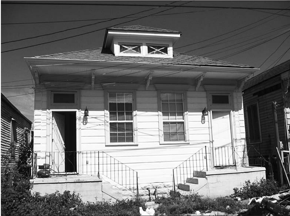
A nearly rehabilitated duplex in the Tremé/Lafitte neighborhoods in Orleans Parish. Photo credit: James Goedert.
