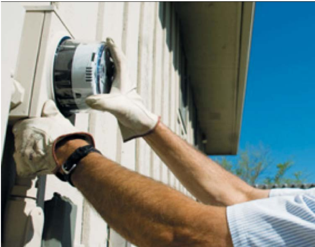
Installation of Smart Meters
