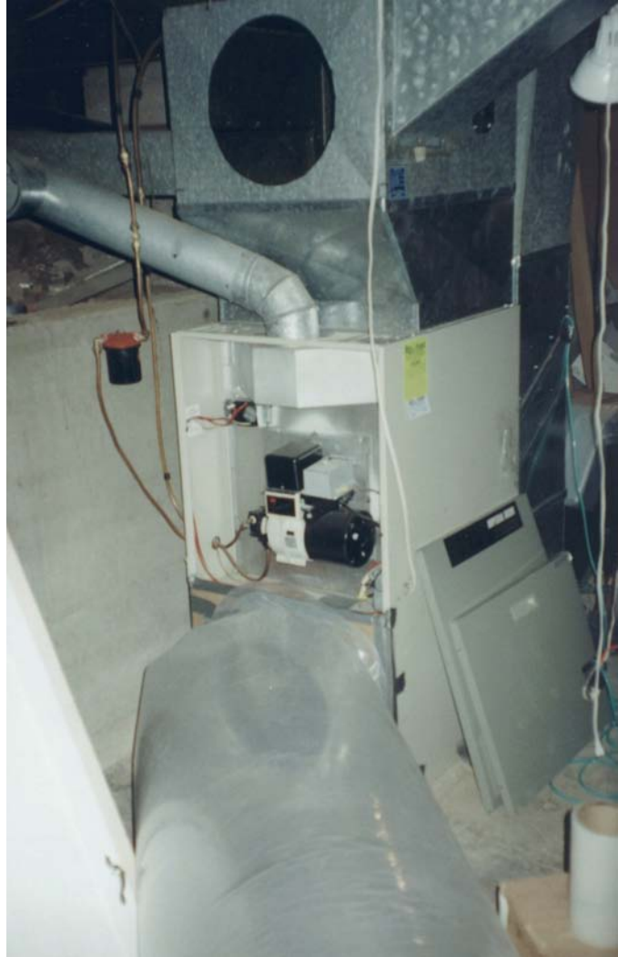
Fig. 2.2. The Aeroseal tubing connection.
