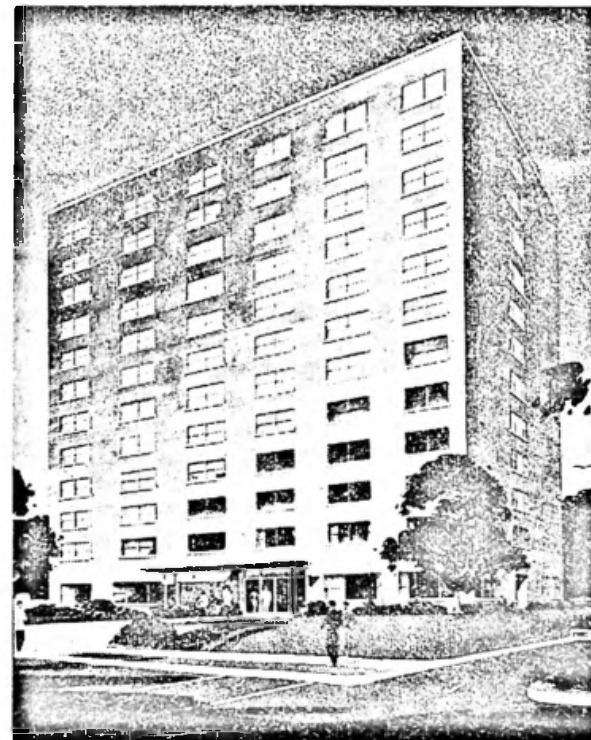
OEA Senior Citizens Apartment Building under construction in Omaha, Nebr., will provide 132 efficiency apartments for retired teachers and other retired persons. The project is sponsored by the Omaha Education Association. A mortgage of $1,144,000 was insured by the FHA under the special Section 207 provisions applying to housing for the elderly.
