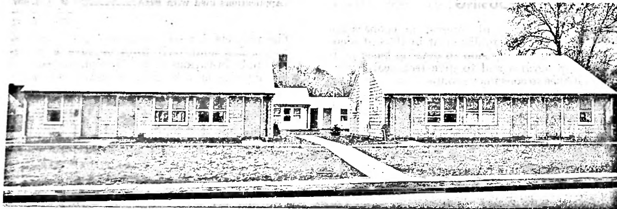
Vine Court, Hartford, Conn., a rental project designed to provide pleasant living for elderly tenants, was financed with a mortgage insured by the Federal Housing Administration under its elderly-housing program. The sponsor was Church Homes, Inc., a nonprofit group representing four local Congregational churches.
