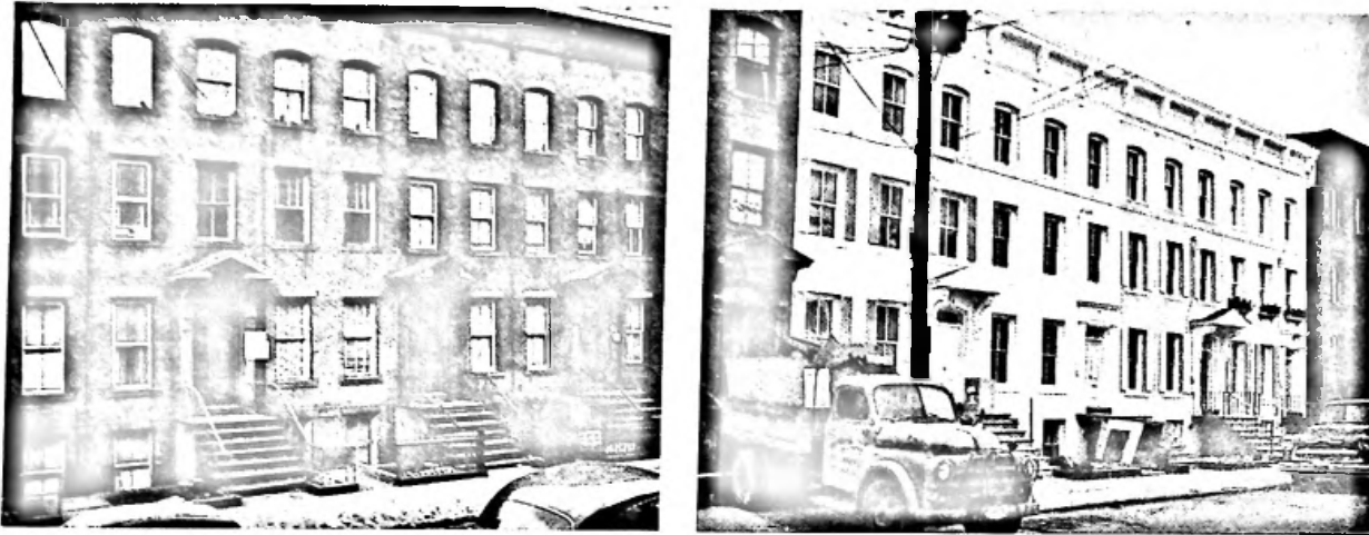
Wooster Square urban renewal project, New Haven, Conn.—Rehabilitation financed with Section 220 FHA-insured mortgages. The two-family houses shown here before and during rehabilitation are priced at $21,000.
