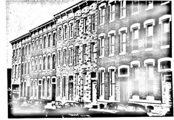
Part of Harlem Park urban renewal area, Baltimore, Md., in which FHA, URA, and the Baltimore Urban Renewal and Housing Agency are cooperating to furnish homeowners with a "one-stop" rehabilitation service.
