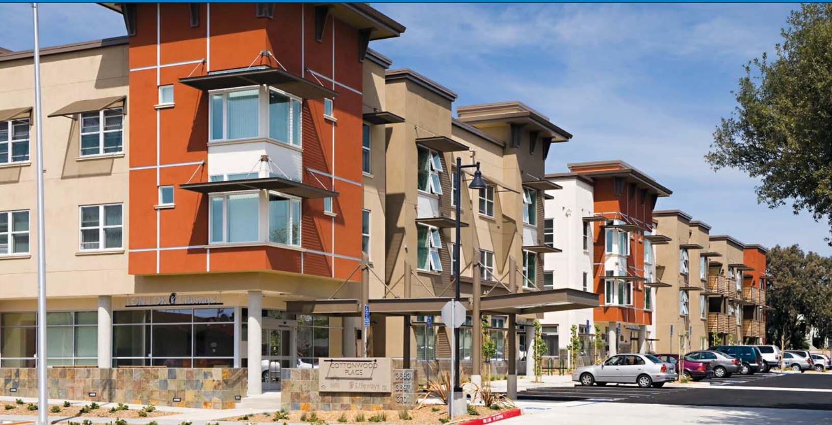
The state of California gives extra points for projects that offer in-unit broadband when awarding low-income housing tax credits. Edén Housing's Cottonwood Place, in Fremont, provides wired access and a modem to each of its 98 units.
