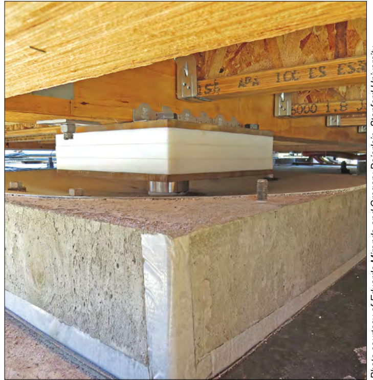
Stanford University engineers developed construction modifications such as a unibody design and seismic isolators that make homes more resilient to earthquakes.
