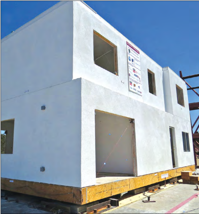
Stanford University engineers developed construction modifications such as a unibody design and seismic isolators that make homes more resilient to earthquakes.
