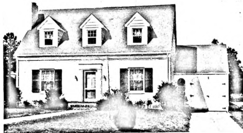
Monthly outlays for this $6,500 Carolina home total $46.30 under the FHA plan. As in the other cases, payments cover all charges.
