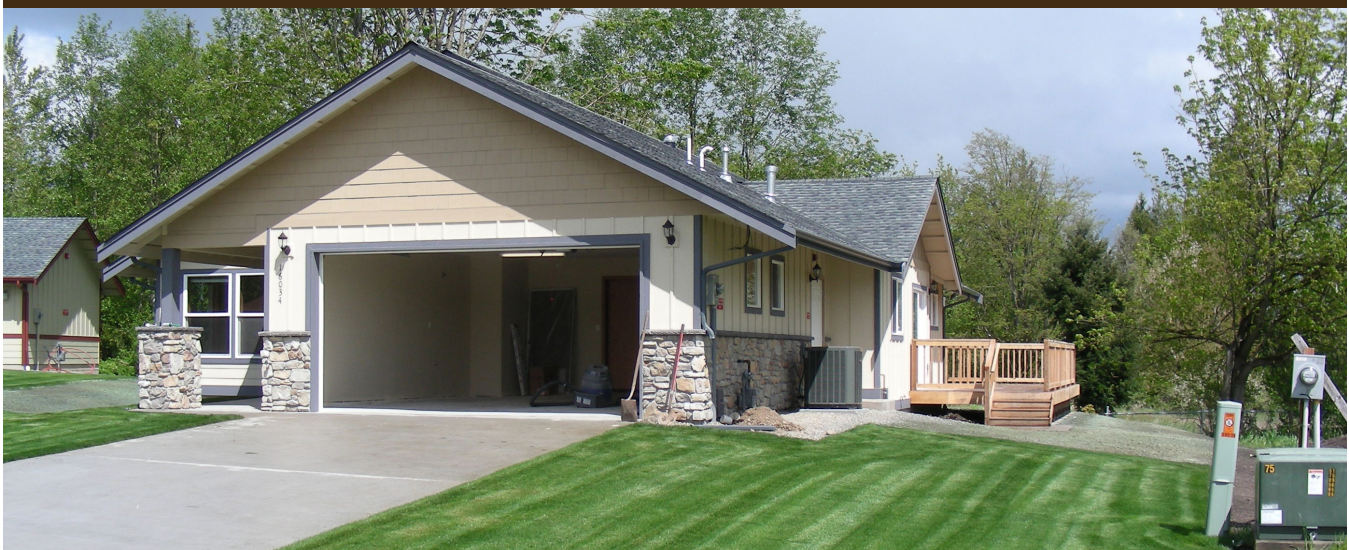
Homes built by the Muckleshoot Indian Tribe in Washington state using funds from the American Recovery and Reinvestment Act of 2009.
