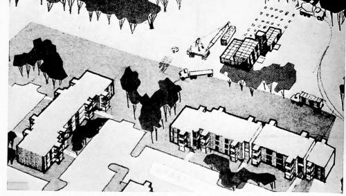
out restrictions. The dimensions selected lend themselves to construction of a unit suitable in size for easy transport. The measurements already constitute a standard in the container industry.
