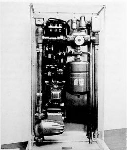
The system is adaptable to hydronic or hot air systems, and it also lends itself to conversion as a cooling element. By providing modified coil units in the plenum chamber of a hot air system with proper antifreeze agents, this system could also be utilized with
