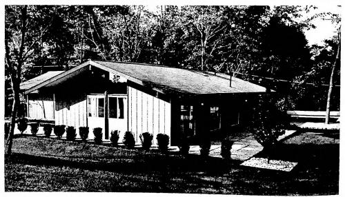
Exteriors of the wall panels are prestained, textured plywoods or hardboards, with masonry veneer available as an option. Interiors are 1/4-in. scarfed plywood, glue-nailed to the framing and covered with seamless, heavy vinyl wall fabric or conventional gypsum board.
