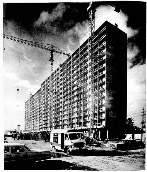
Bathroom and kitchen modules are not part of this system, but such modules can be incorporated easily because of the precise nature of the system itself. Pines, conduits, and utility boxes are fastened to the forms and cast in the concrete walls and slabs. All duct openings are framed out without weakening the basic structure. Conventional foundations are specified and location can be on a wide variety of soil conditions.
