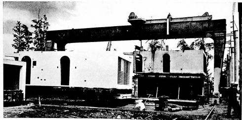
No specific architectural constraints or design arrangements are required by the system. Conventional interior work, standard plumbing, electrical, and heating/air conditioning facilities are planned, usually to be installed at the factory to reduce costs. Because the system is lighter than conventional construction, it is more adaptable to various soil conditions. The system is suitable for almost all terrains. The only requirement is that there must be access for the erecting crane.
