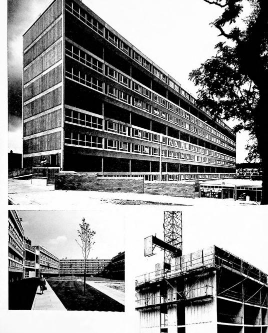
Forms are used to build open-ended structures, so that the forms or combinations of them can be pushed through from one side of the building to the other as the concrete cures. Facade openings can then be filled in with almost any desired nonbearing material, from masonry to glass window walls or sandwich panels of traditional materials. Prebuilt reinforcing cages are placed as soon as the forms are in position, eliminating site work. Foundations for the structures are conventional.
