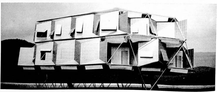
the unusual structural system. Fastening is accomplished through deformation of each end of the identical 13-ft. (4-in. diameter) lengths of tubing, these flattened ends thus mating securely with the slots in the hub. The structural system resulting from such an assembly of tubing and flooring panels is capable of supporting itself and concommitant housing live loads up to five stories high.
