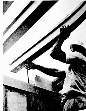
The panel-and-post system produces a board-and-batten effect for both exterior and interior wall surfaces, which may be easily painted and are virtually maintenance free. The extruded shapes for the roof system results in an attractive beam ceiling effect. No wood or plastic trim is used throughout the house; the entire structure is decay and termite proof, has good sound isolating characteristics, and is resistant to hurricane-force winds.
