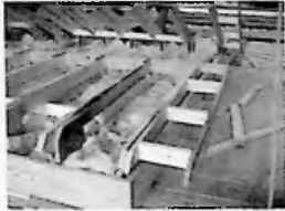
Fig. 3.22 Unfolded roof rafters showing attic insulation
