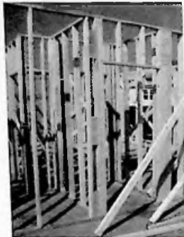
Fig. 3.60 Exterior panels set and braced plumb
