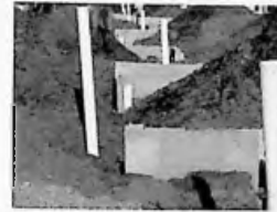
(B) Underslab services at foundation offsets
