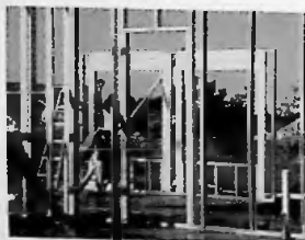
Fig. 3.80 Step 6: Panels are plumbed and braced
