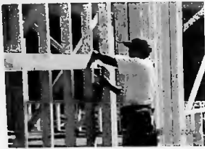
Fig. 3.88 Field installation of blocking for horizontal OSB pattern
