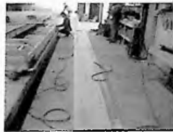
Fig. 3.17 Overall view of box girder with layout marks
