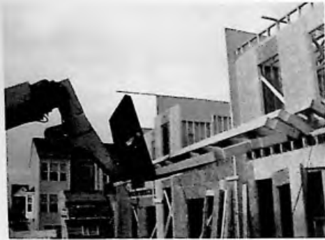
Fig. 3.39 Preengineered component handling
