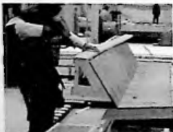
Fig. 3.26 Attaching folding overhang
