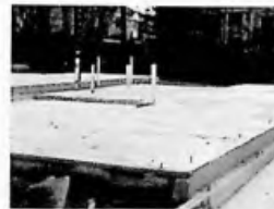
Fig. 3.35 Underslab plumbing and finished slab
