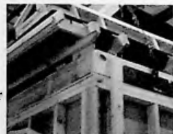
Fig. 3.31 Mating roof assembly to wall assembly
