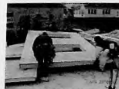
Fig. 3.58 Manual sorting of panels
