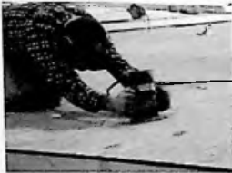
Fig. 3.23 Routing roof sheathing to accept hinges for drop-in panel
