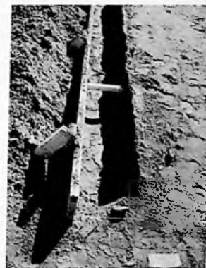
Fig. 3.72 Formwork, stakes, hand-dug foundation trench
