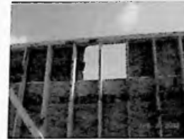
Fig. 3.66 OSB partially removed from outside of wall panel
