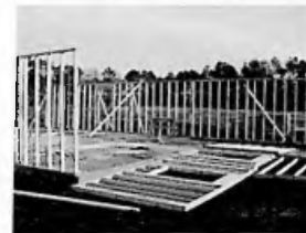
Fig. 3.85 Panels arranged for scribing anchor bolt locations
