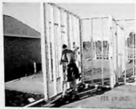
Fig. 3.78 Step 4: Panel is placed over anchor bolts
