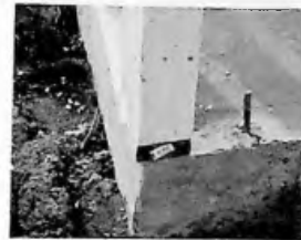
Fig. 3.83 Panel end, chalkline, and anchor bolt
