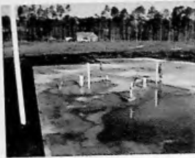
Fig. 3.74 Completed slab with utility risers
