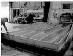
Fig. 3.18 Installation of ceiling joist/kneewall/rafter assembly
