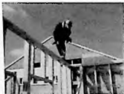
Fig. 3.61 Panels aligned by nailing to top plate
