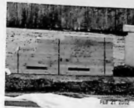
Fig. 3.81 Wall panels delivered to site
