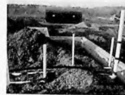
(A) Underslab services placed prior to backfill and gravel
