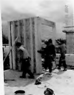
Fig. 3.59 Interior and exterior panels set and braced plumb
