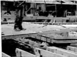
Fig. 3.24 Drop-in panel ready for sheathing
