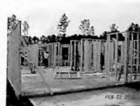
Fig. 3.86 Exterior panels braced plumb, interior panels being set
