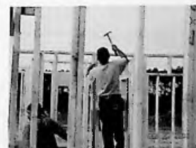
Fig. 3.87 Aligning panel top plates
