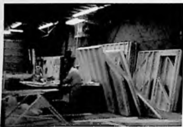
Fig. 3.14 Dormer panels fabricated from "cut sheets"
