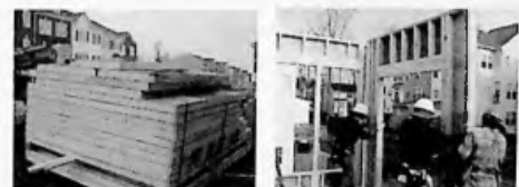
Fig. 3.37 Wall panels as delivered and installed
