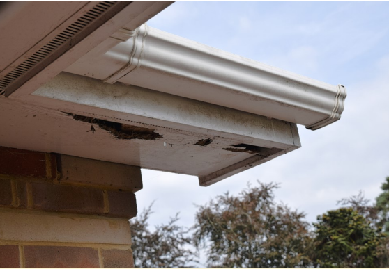
Damaged soffit.
