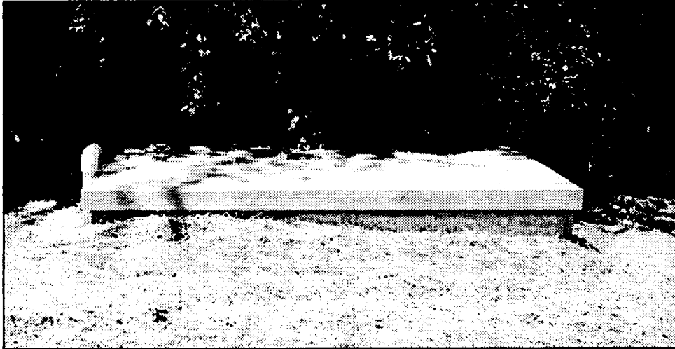
Photo 1: Typical Sand Filter Extending Above Grade
