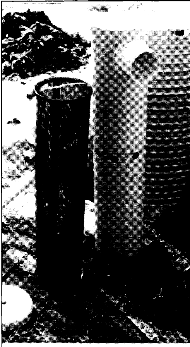
Photo 9: Filter Used at Outlet of First Chamber of Septic Tank
