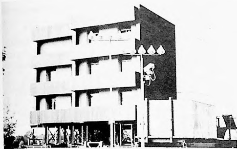
G. Top Three Floors Complete—Building Being Raised for Installation of Next Floor
