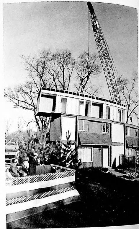
F. Module placement using mobile crane
