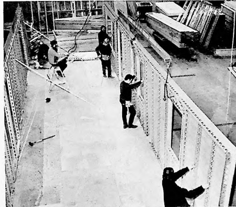
J. Factory assembly of Alumiframe wall panels.
