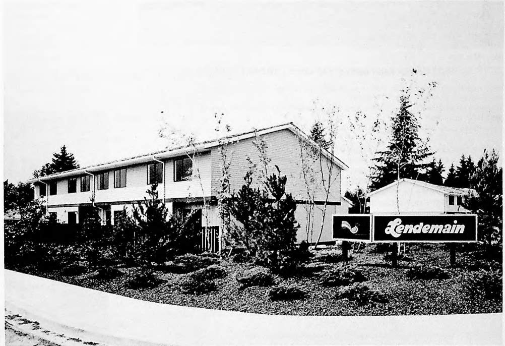
L. Completed ACSI Townhouse units at King County prototype site.
