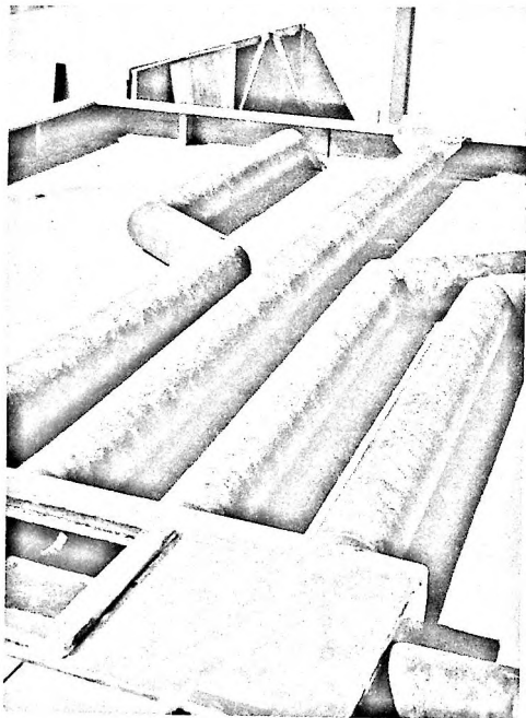
B. Ducting in place between two-story townhouse shells.
