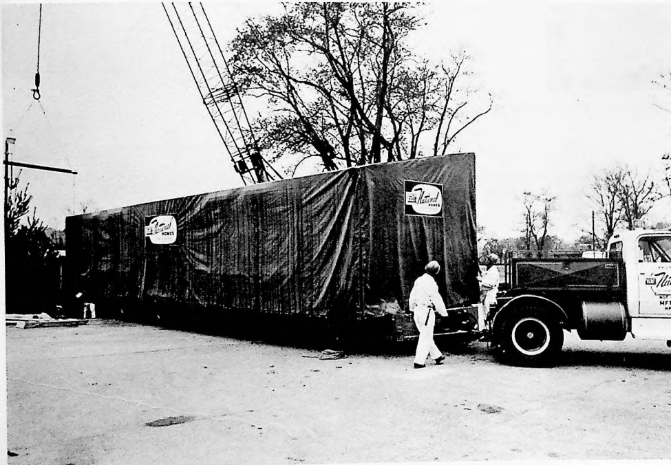
G. Module readied for lifting from trailer
