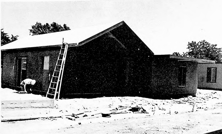
K. Fiber-Shell panel house, Belen, New Mexico.
