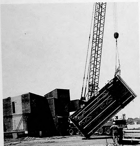
I. Field erection of tower module
