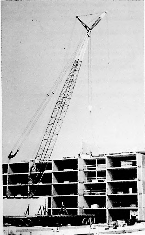
N. St. Louis prototype erection under progress
