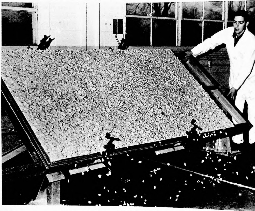
I. Excess stone is removed from structural panel before curing.
