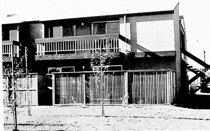
M. ACSI Garden Apartments at Sacramento BREAKTHROUGH site.
