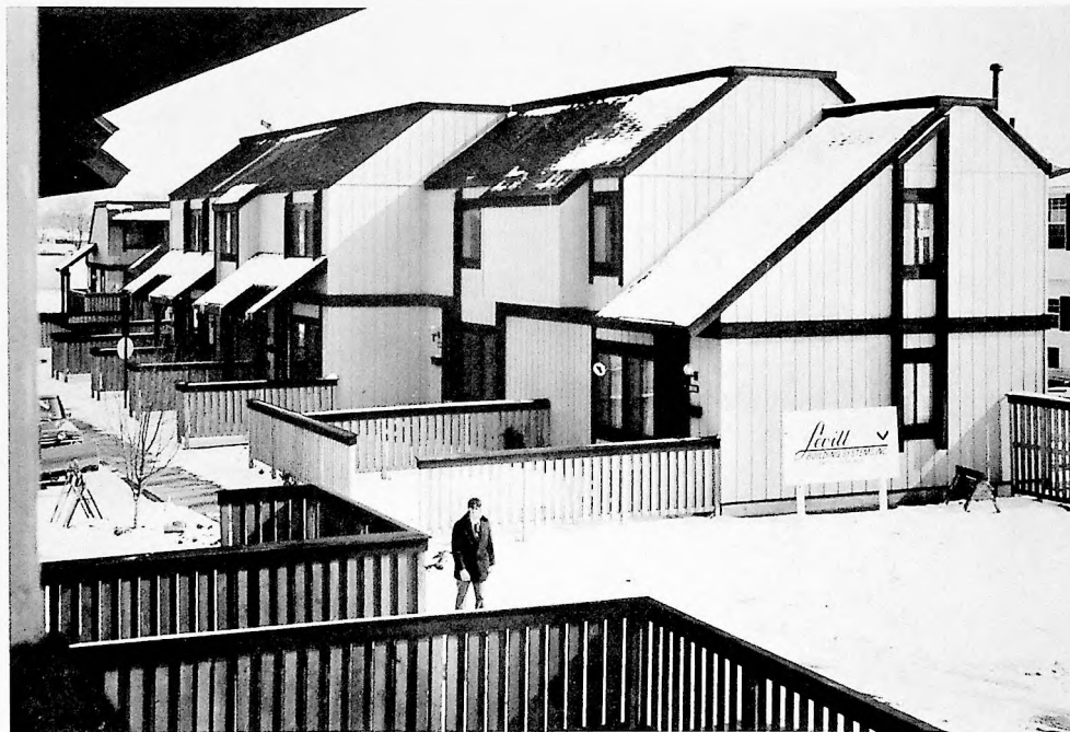
F. Considerable architectural variety is offered by Levitt townhouses.
