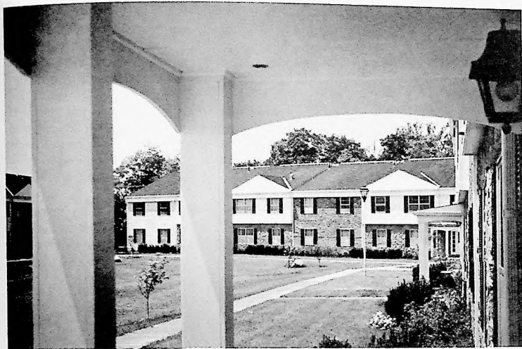
I. Colonial style is prevalent at Scholz' Columbus, Ohio project
