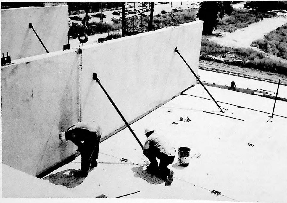
M. St. Louis prototype wall and slab erection.
