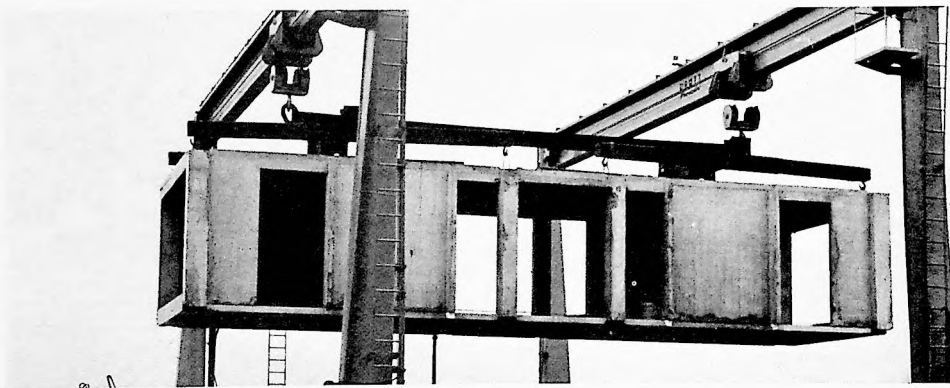
M. Factory-Cast Structural Concrete Box Module On Specially Designed Crane
