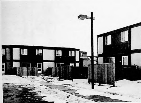
L. National Homes Operation BREAKTHROUGH housing - Kalamazoo, Michigan
