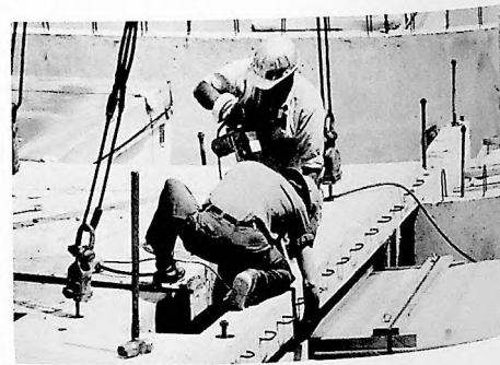
H. Floor panel installation
