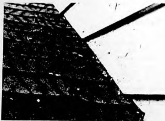
A second layer of shingles has filled the former gap between roof and siding, causing the siding to deteriorate.
