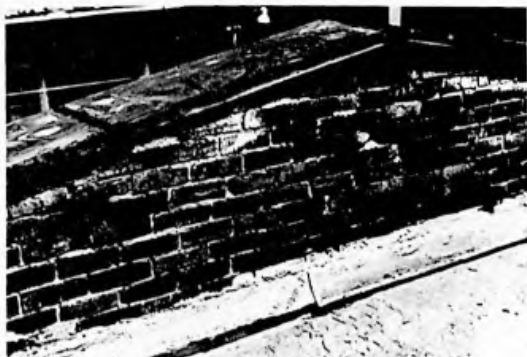
A deteriorated parapet wall that badly needs repointing. Fortunately, the wall has not yet exhibited serious movement, but will if left unrepaired.
