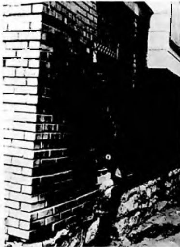
An extreme case of structural failure in a masonry wall due to foundation settlement. The wall and foundation must be completely rebuilt.
